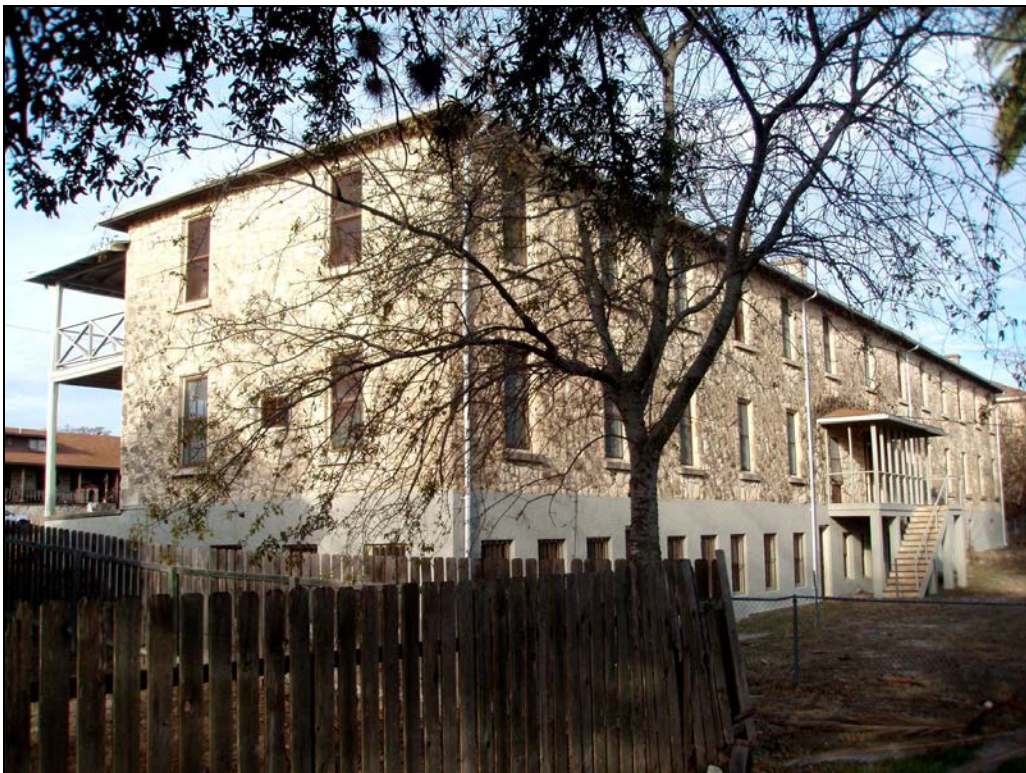
New Cavalry Barracks, Fort Clark, Texas back corner [East] elevation.
