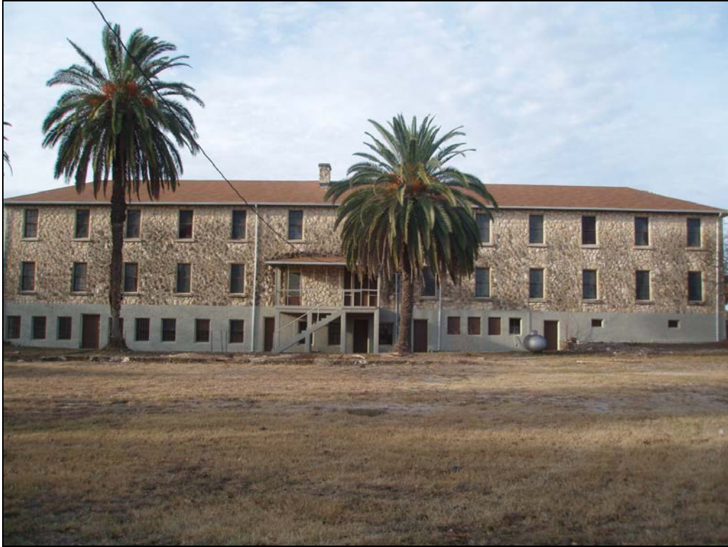
New Cavalry Barracks, Fort Clark, Texas back [Northeast] elevation.
