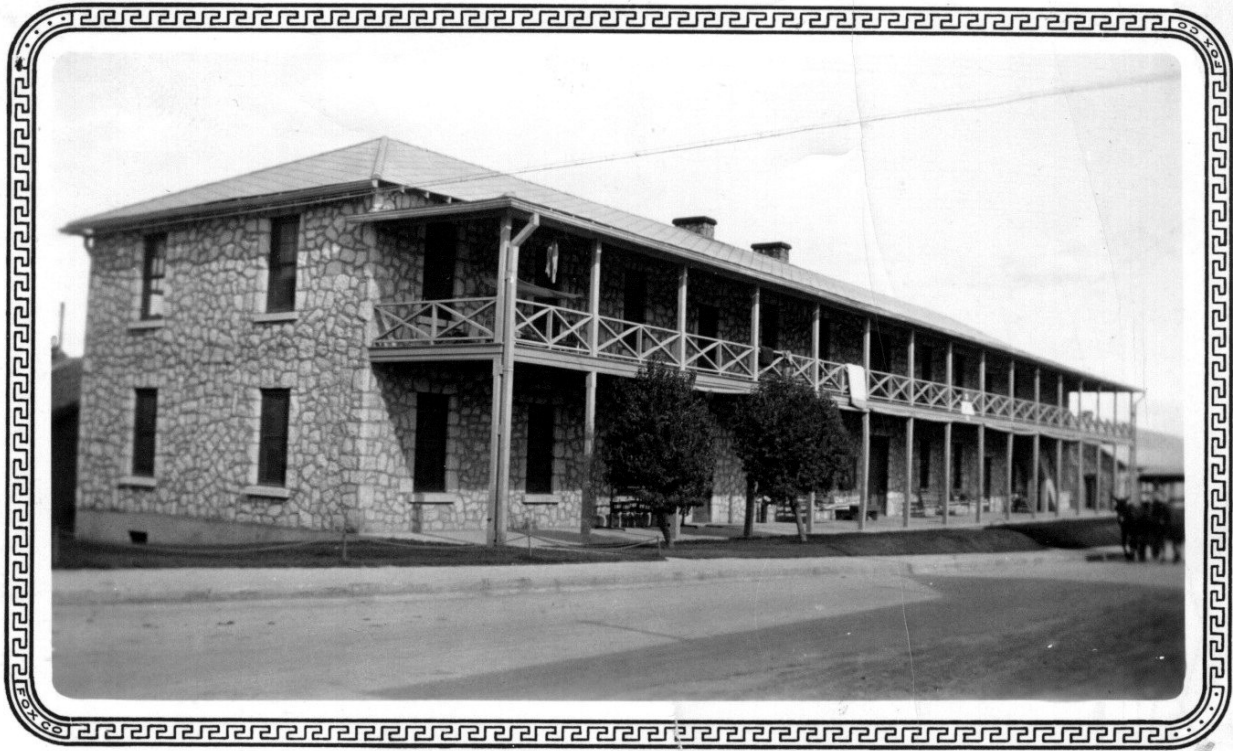
New Cavalry Barracks building, Fort Clark, Texas circa 1932
