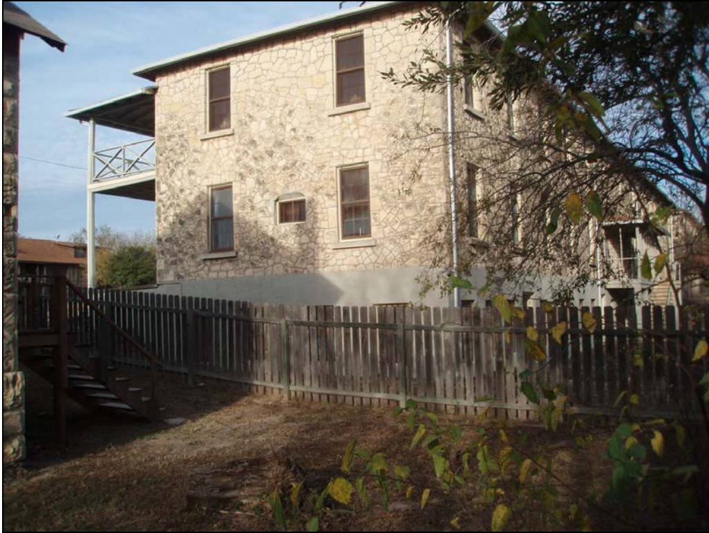
New Cavalry Barracks, Fort Clark, Texas side [Southeast] elevation.
