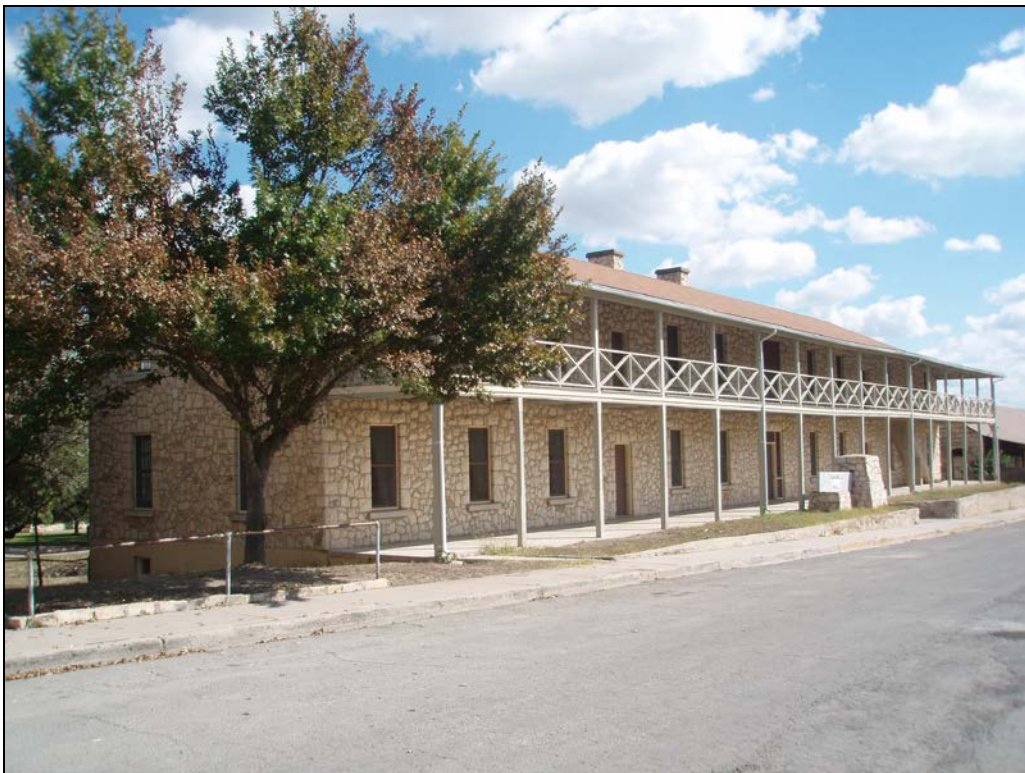
New Cavalry Barracks, Fort Clark, Texas front corner [West] elevation.
