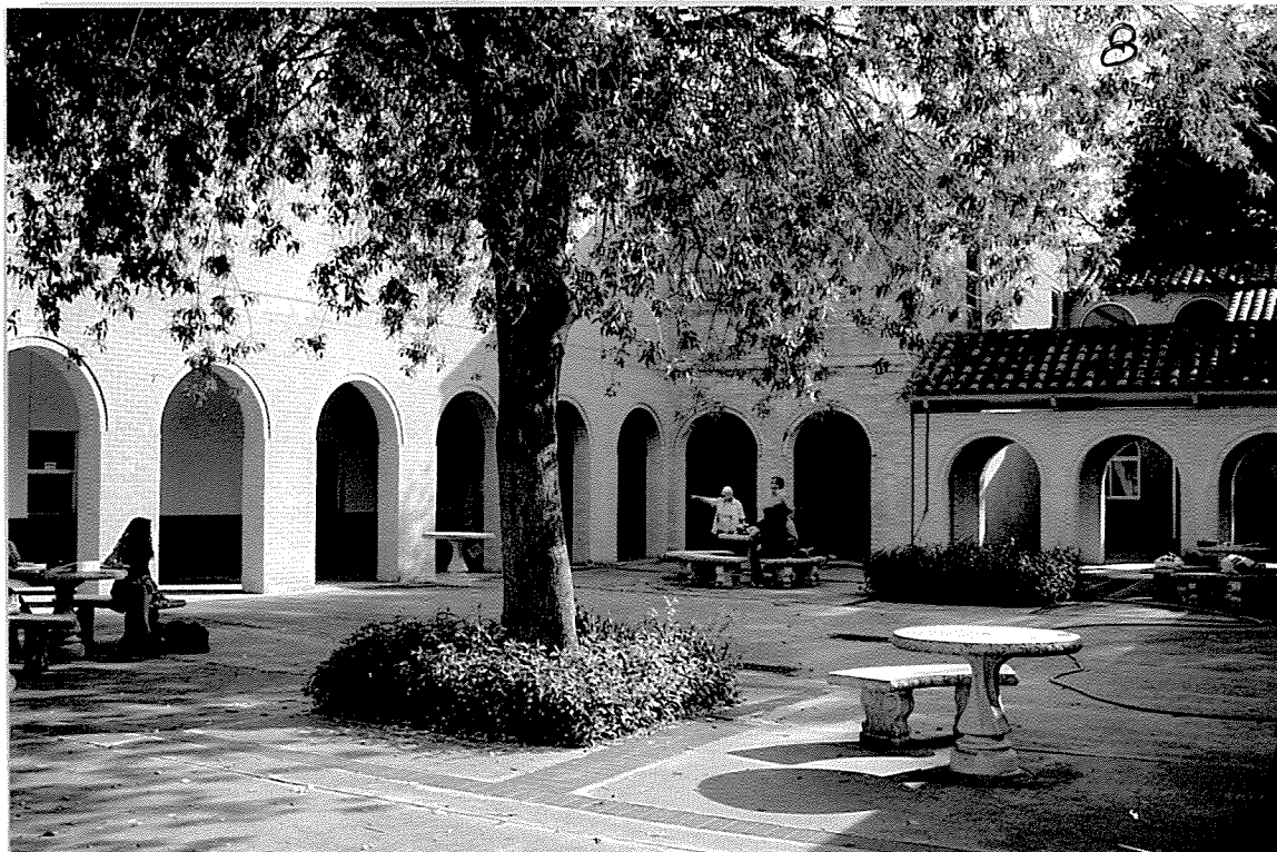
8. East side with patio, north side of arcade at right
