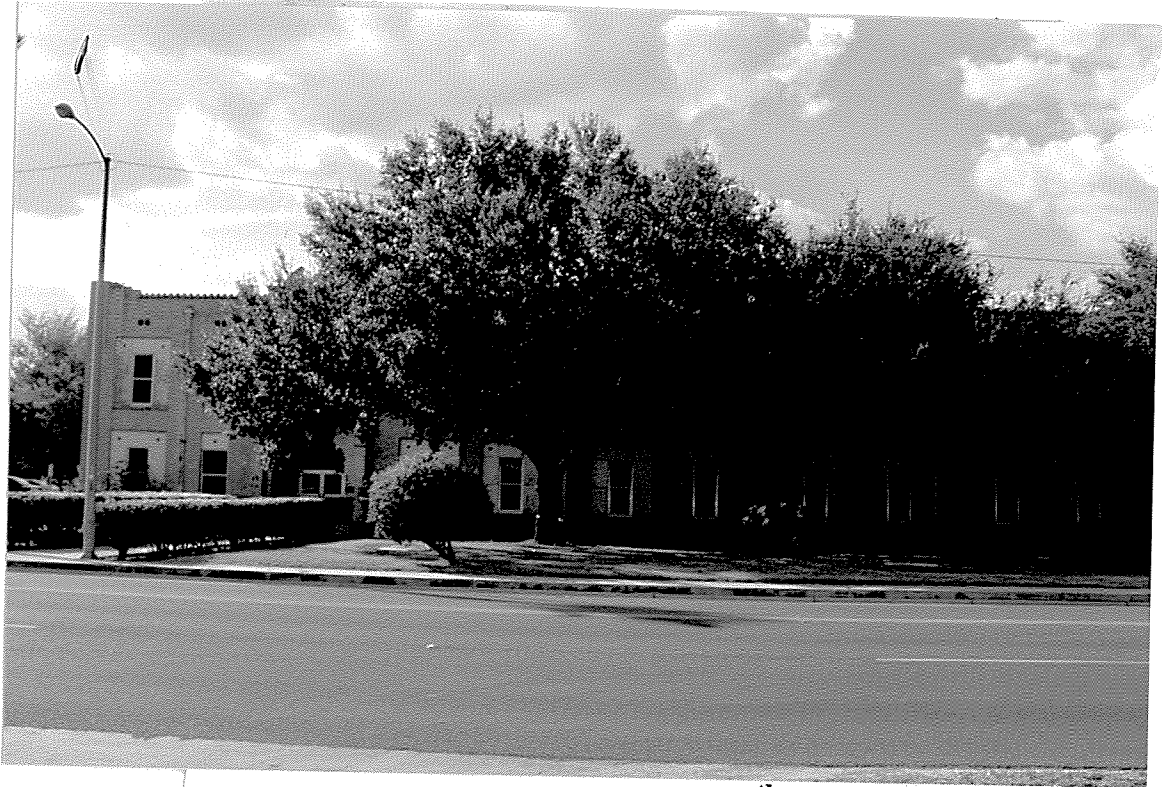
1. West façade from across 10 th Street
