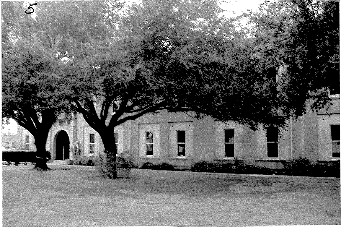
5. West façade, looking east from 10 th Street
