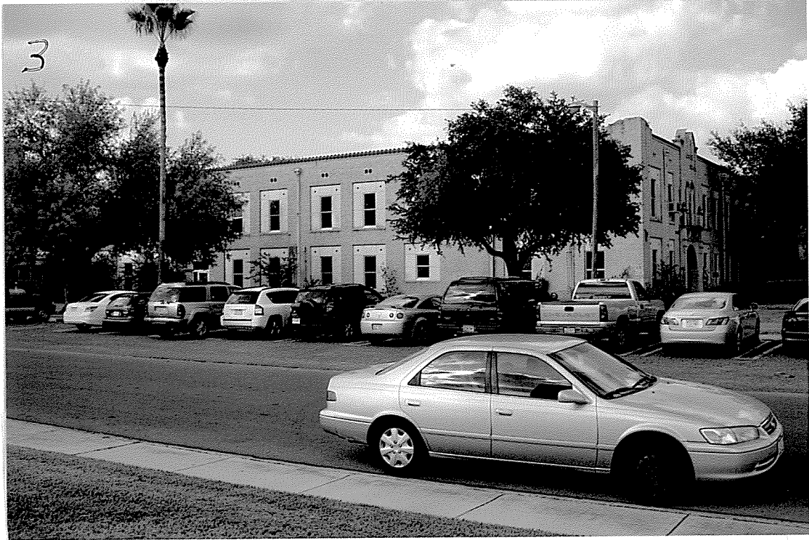
3. South side from across Jasmine Street, looking north
