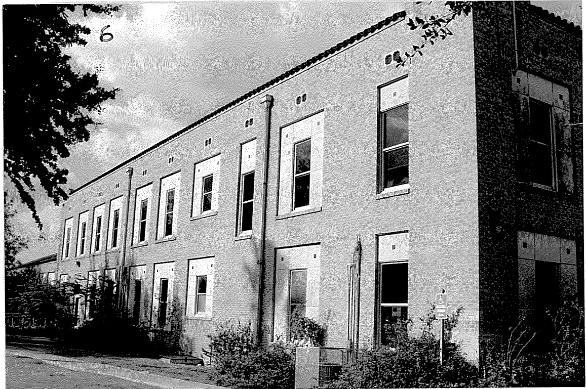
6. South side, looking north from Jasmine Street
