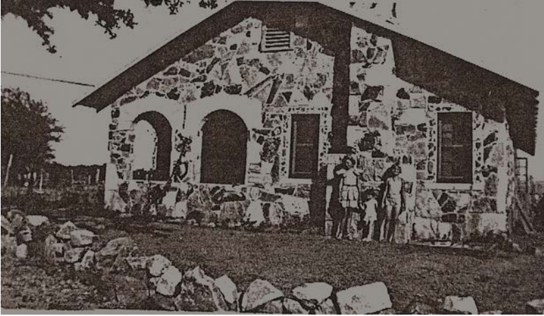
Fig. 1 – showing historic double hung windows.
