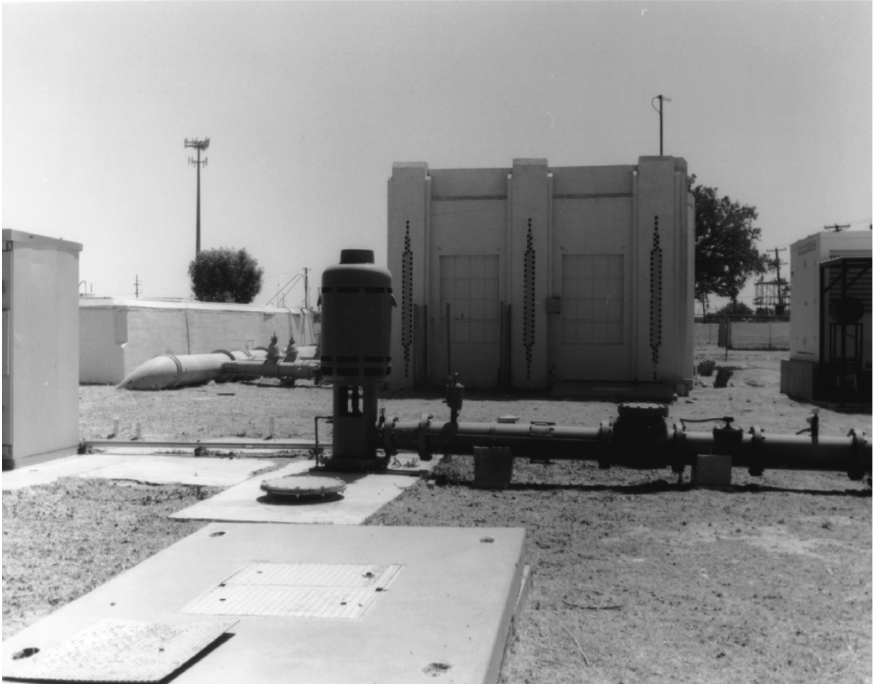
Photograph 6. West façade, camera facing east. Photograph by H. Gregory Quinn.
