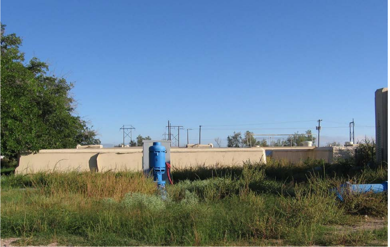
Figure 8. West-most settling basin in foreground, east-most settling basin at right, camera facing north. Photograph by Summer Chandler.
