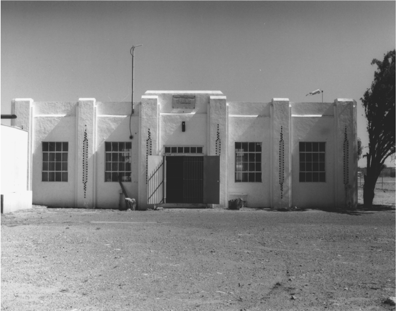
Photograph 1. South (front) façade of main building, camera facing north. Photograph by H. Gregory Quinn.
