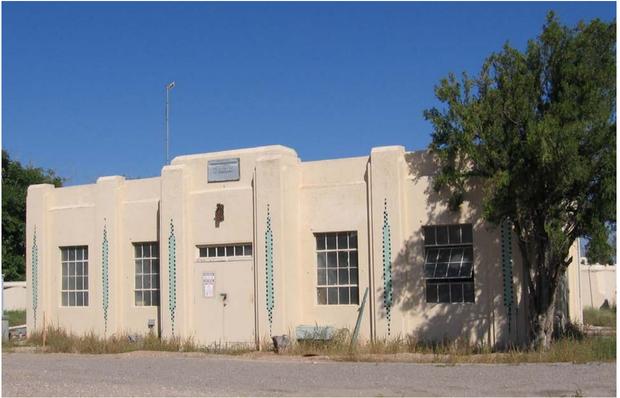
Figure 3. Main (south) façade of the main building, camera facing northwest. Photograph by Lannie Ethridge Kittrell.
