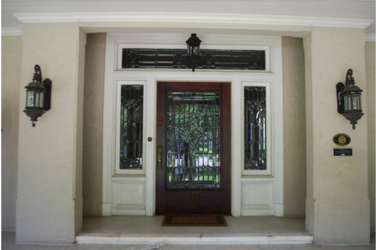
Detail of front door, three quarter sidelights and transom
