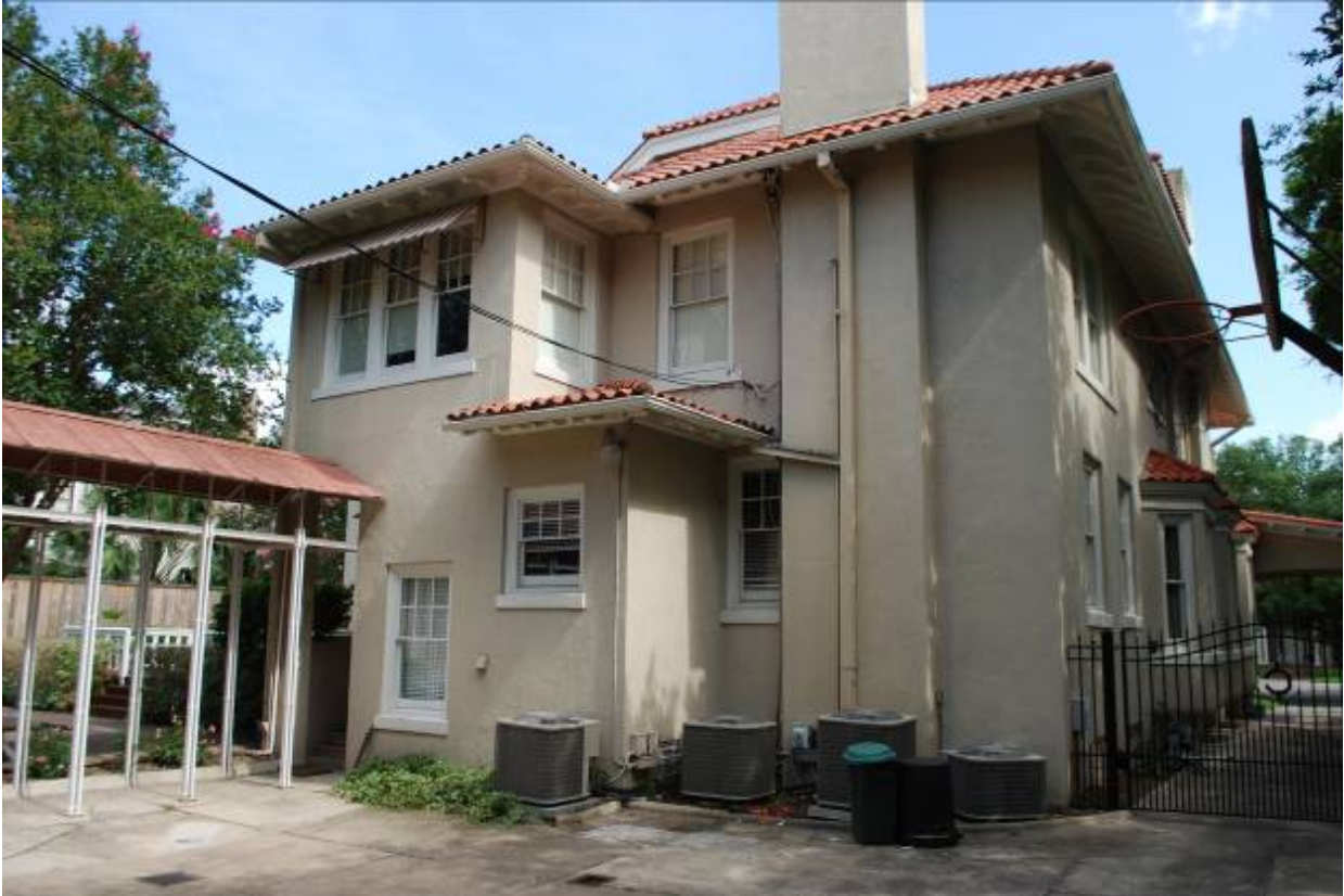
North and west elevations, view south
