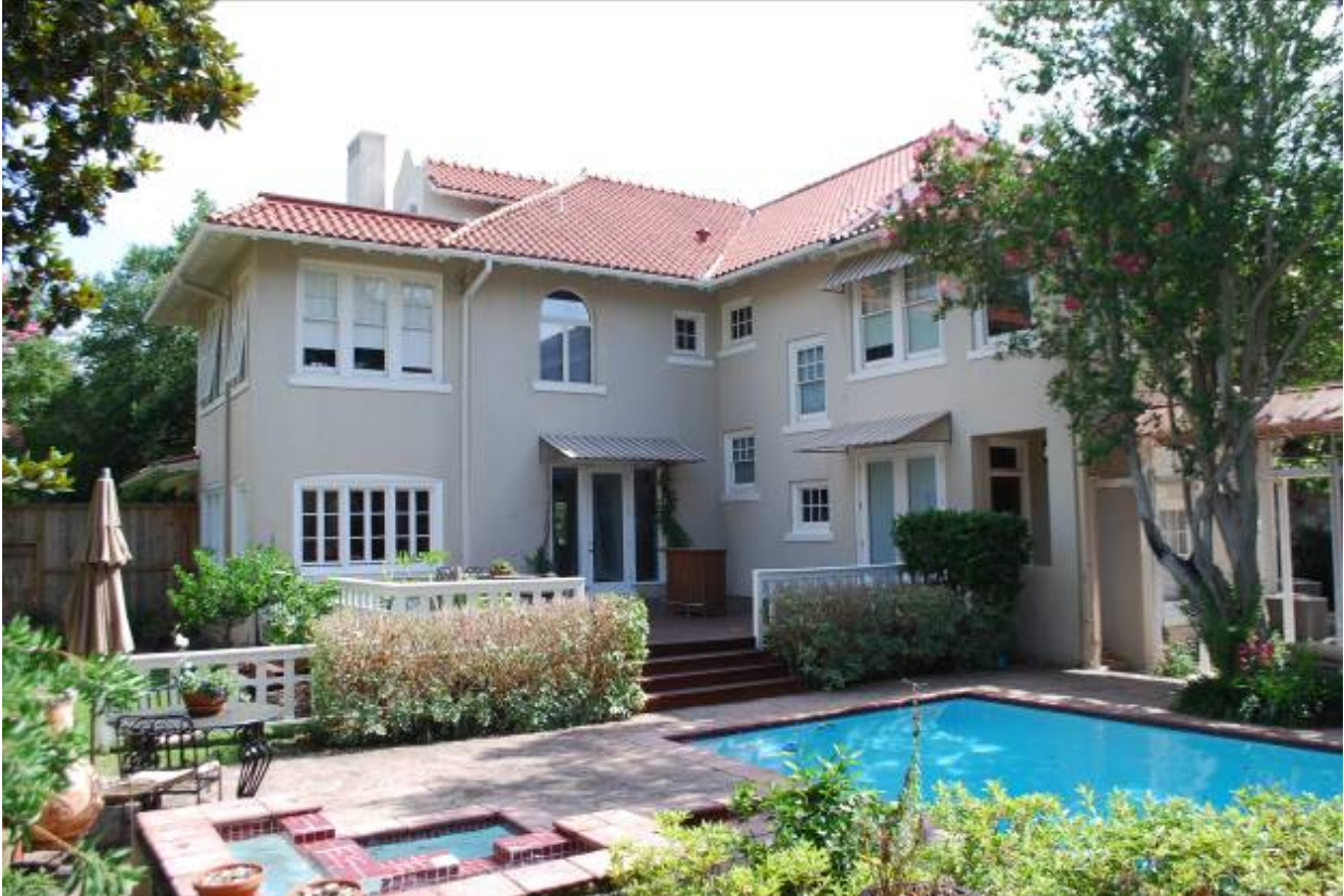
East and north elevations, view south
