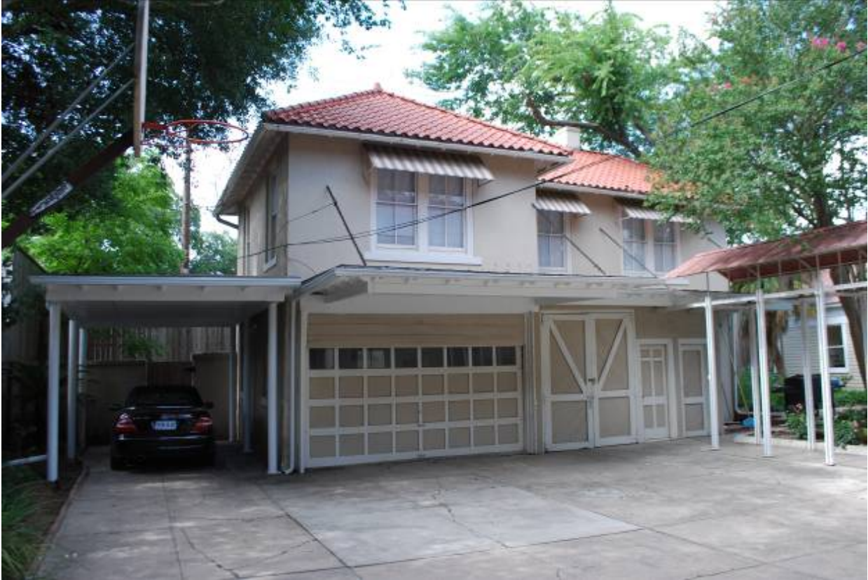
Garage, view north
