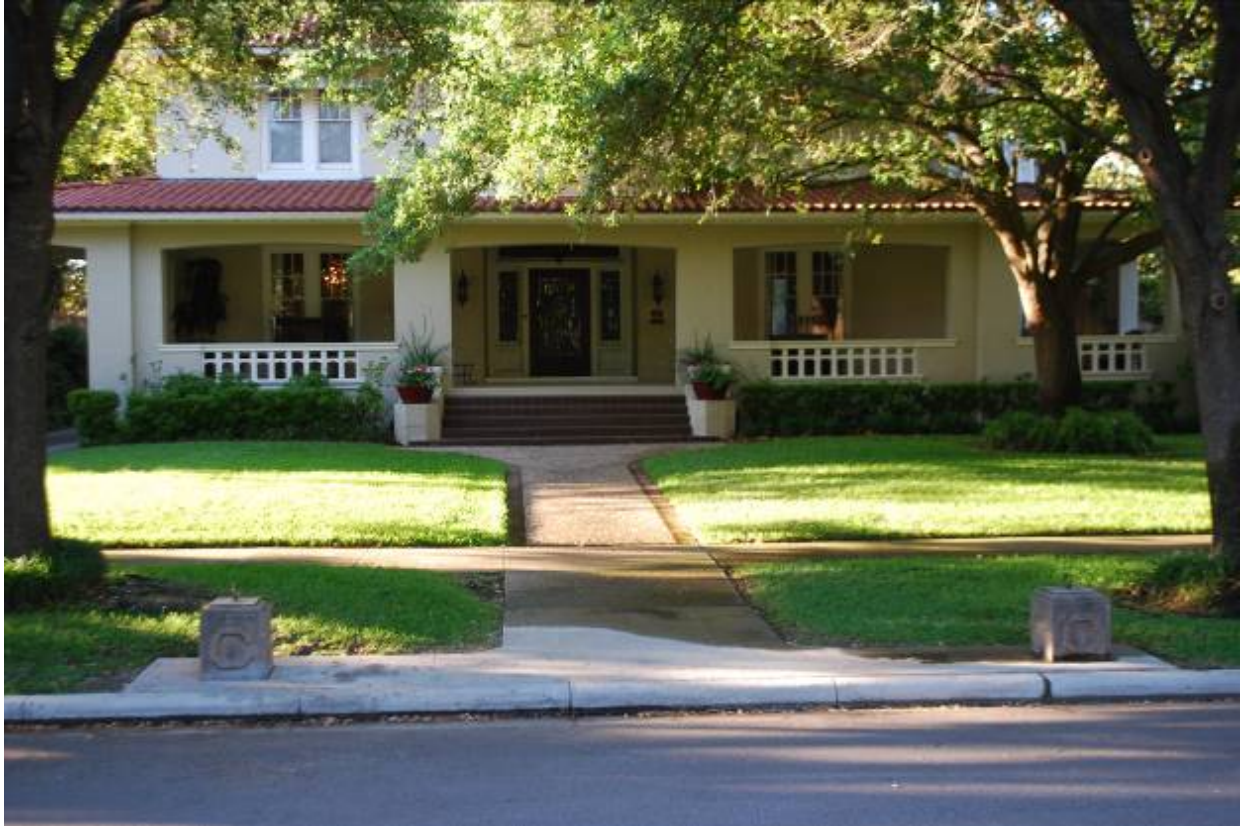
Detail of south façade, front door and hitching posts
