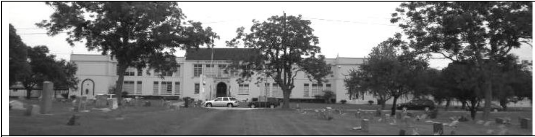
North façade of Main Building (1928) and East and West Wings (1937) taken from the Hill of Rest Cemetery across Market Street from Lee with camera facing south
