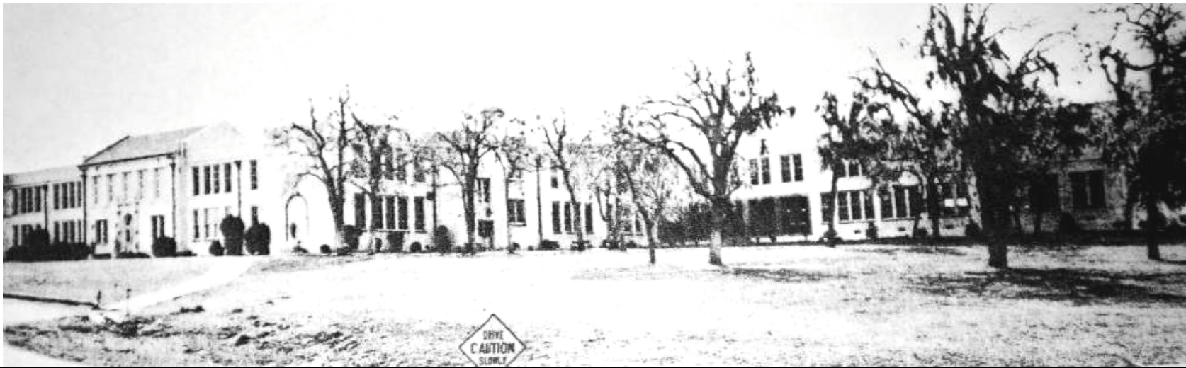
North and west façade of Main Building (1928) with north façade of West Wing (1937) on right from 1940 yearbook with camera facing southeast
