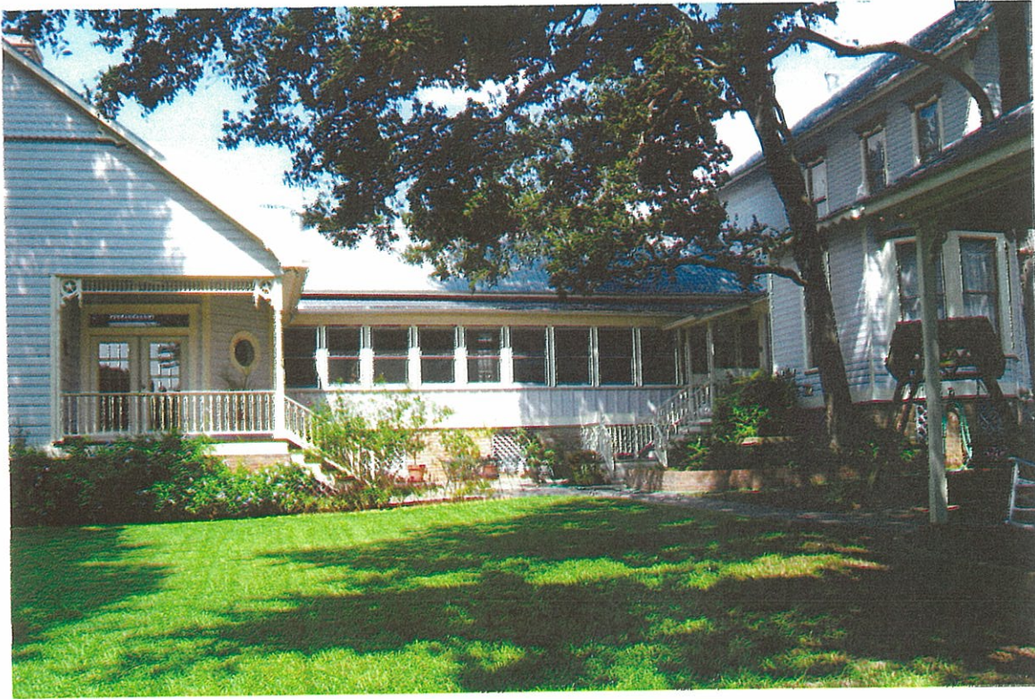
South side - showing the 1995 add-on on the left side of the picture.
