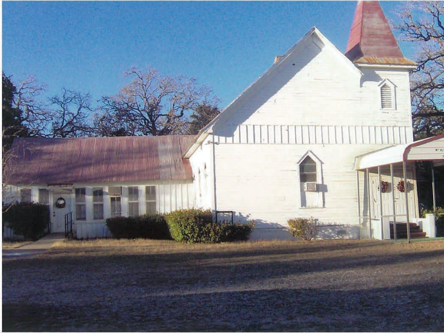
FRONT VIEW OF THE CHURCH—2007 Mt Olive Baptist Church
