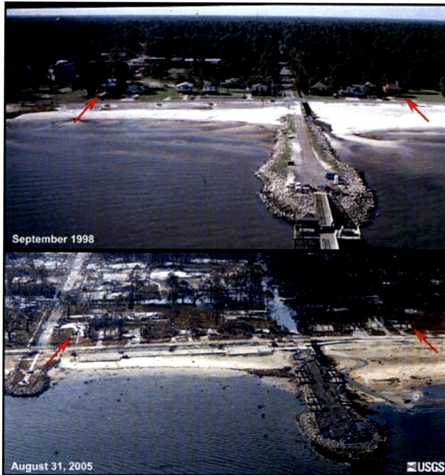
Figure 3. Waveland, MS Katrina Damage
