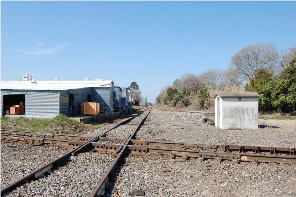
Figure 8: BNSF Galveston Subdivision Crossing in Brenham
