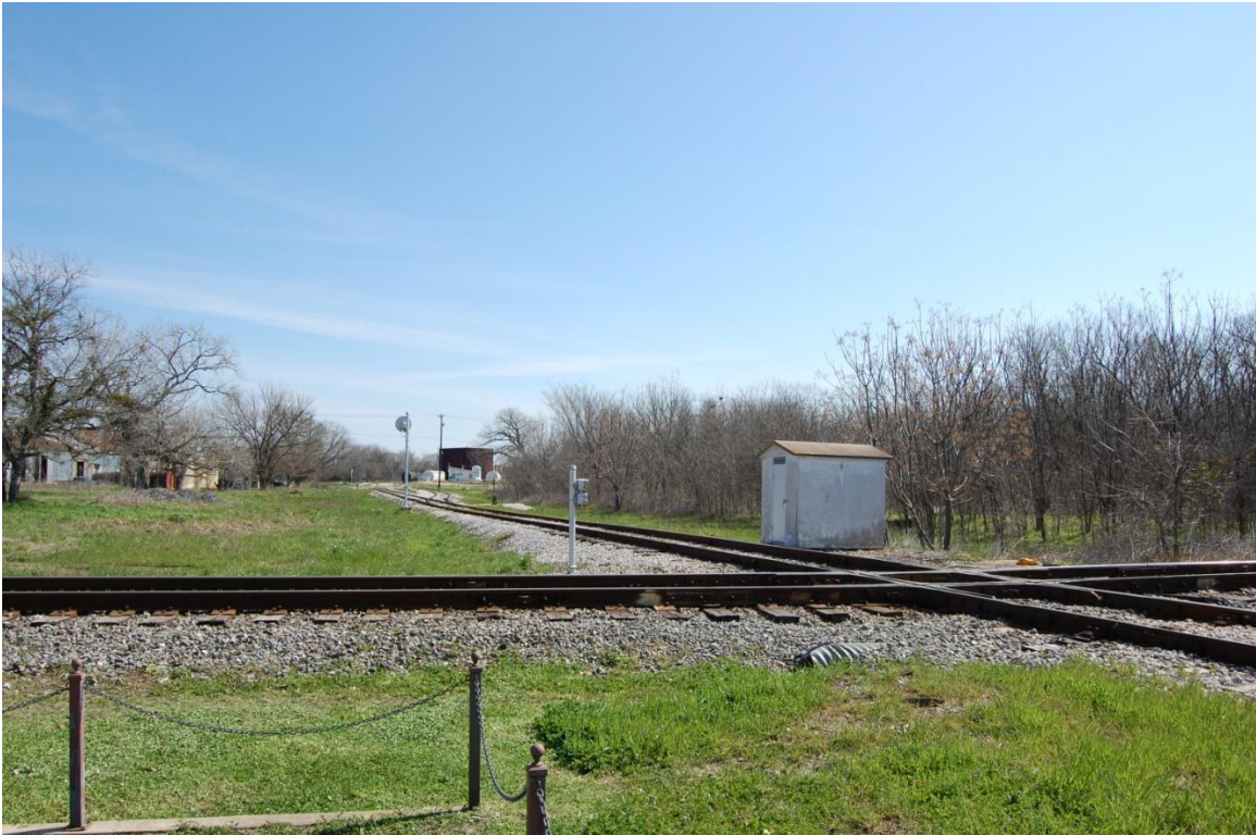
Figure 6: Waco Subdivision Crossing in Elgin
