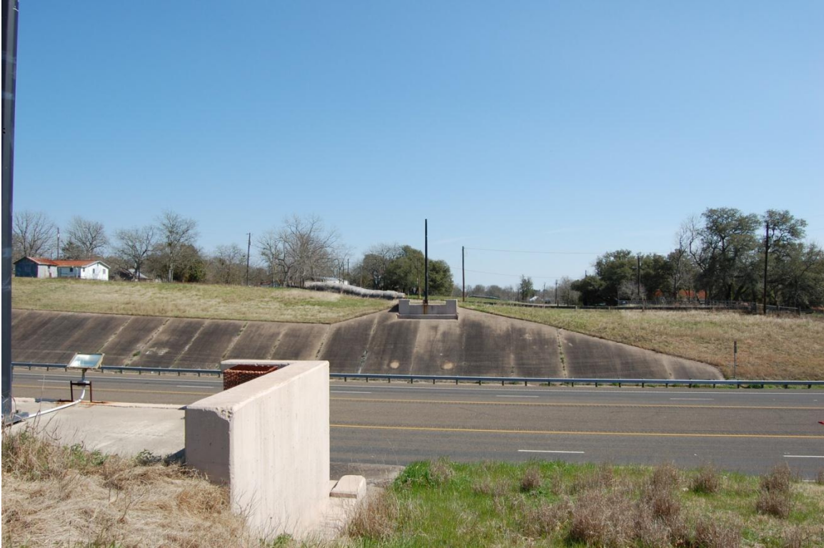
Figure 15: Location of Removed Rail Bridge at U.S. 290 in Burton
