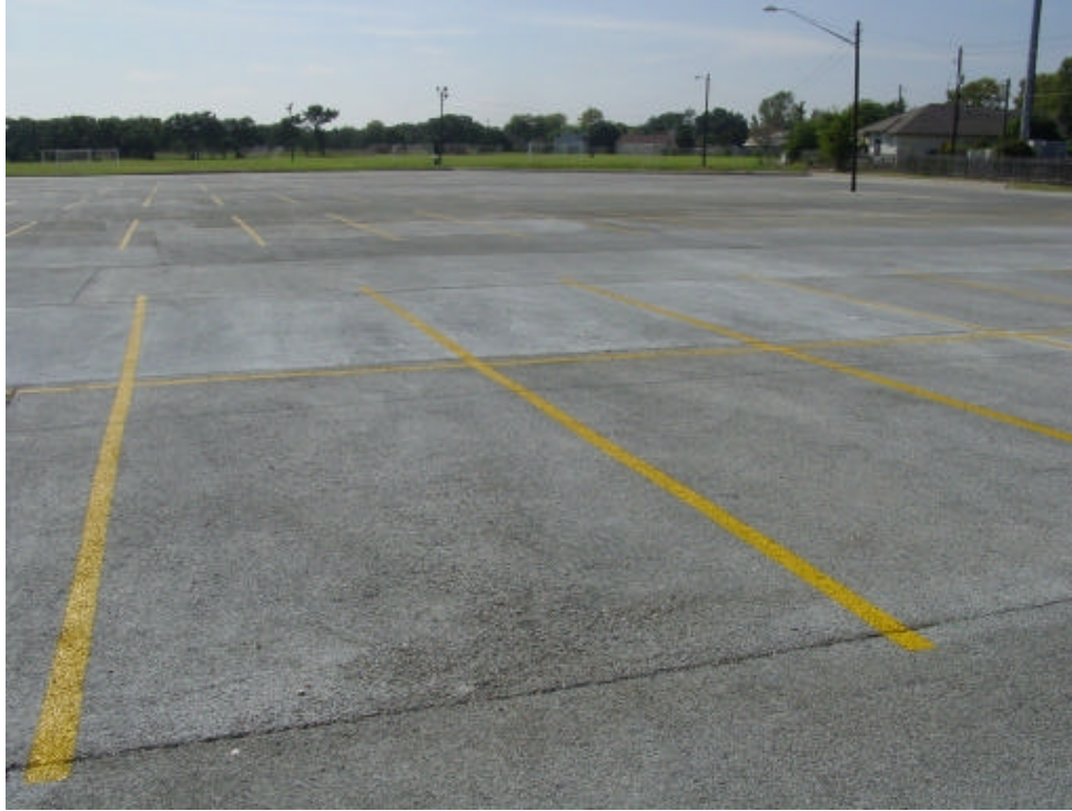
Figure 3-9 Permeable Concrete in Parking Lot at a Recreational Center
