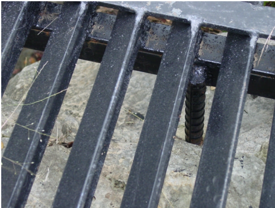
Figure 5-3 Example of Anchor Rebar
