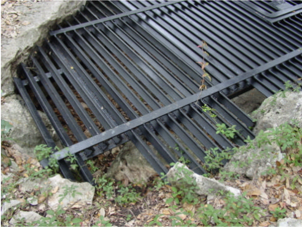
Figure 5-2 Mammal Access Portals Along Edge of Gate
