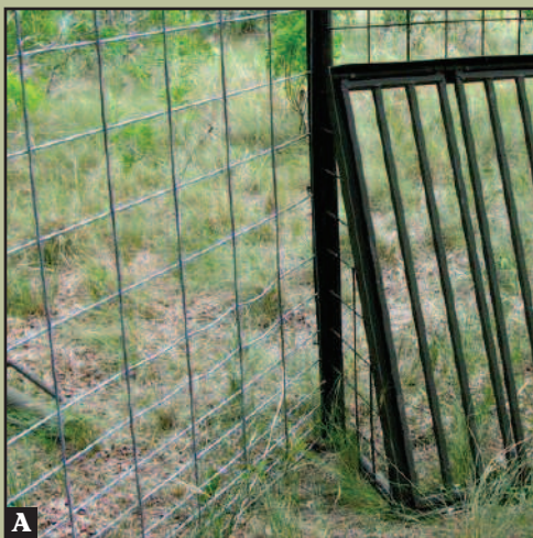
A panel secured to a head gate T-post with doubled wire (A). The remaining panels are attached to one another. It is important to overlap the ends of the panels (B).
