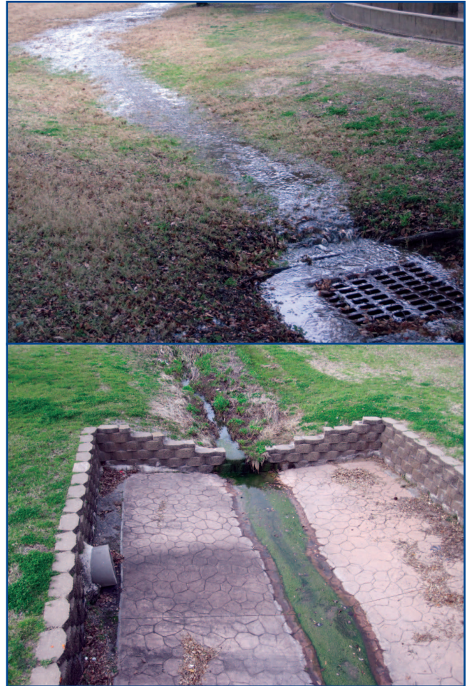
Figure 2. Non-Point Source Pollution: Runoff from roofs, pavement, and even lawns (top) can pick up pollutants that lead to storm drains. As an example, excessive nutrient runoff can lead to algae growth in water bodies (bottom).
