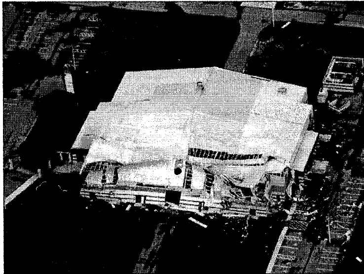
Figure 1: Turner Agri-Civic Center Damage Caused by Hurricane Charley [7]
