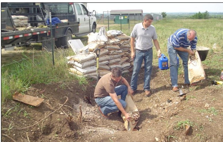
(left to right) Justin Mechell (TAES), Ryan Gerlich (TAES), and Dirk Aaron (Clearwater UWCD), Abandoned Water Well Plugging Demonstration coordinated with Clearwater UWCD (Bell County), June 2009. Photo courtesy of Dirk Aaron (Clearwater UWCD)
