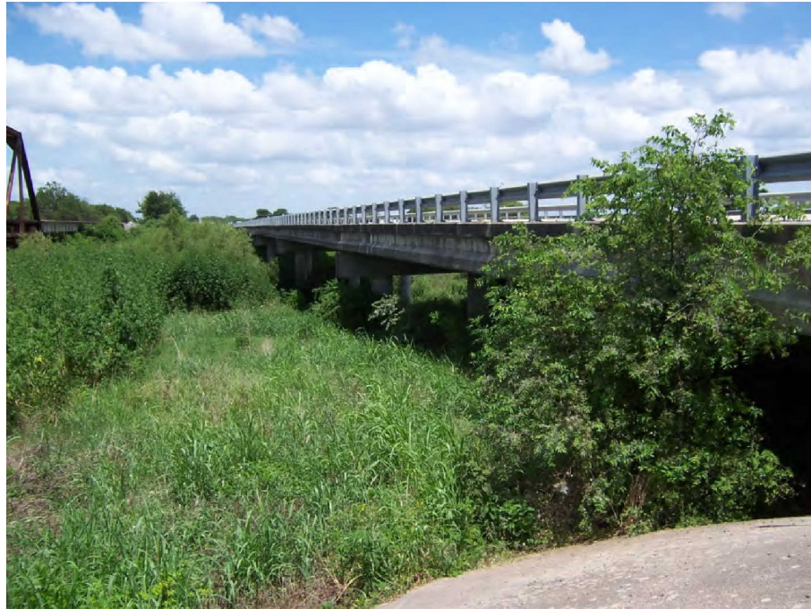
Figure 1.0 – Seco Creek at Hwy 90 Westbound
