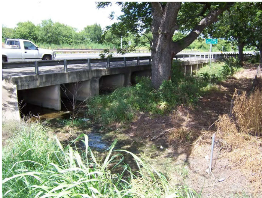
Figure 2.0 – Parkers Tributary at Hwy 90 Eastbound
