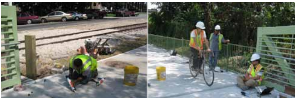
(Left) A worker seals the saw cut where a wire for the traffic counter was installed. The wire senses the presence of bicyclists, and the wooden pole next to the concrete path counts all trail users by direction. (Right) Workers test the traffic counter equipment by riding a bicycle through the sensor area.
