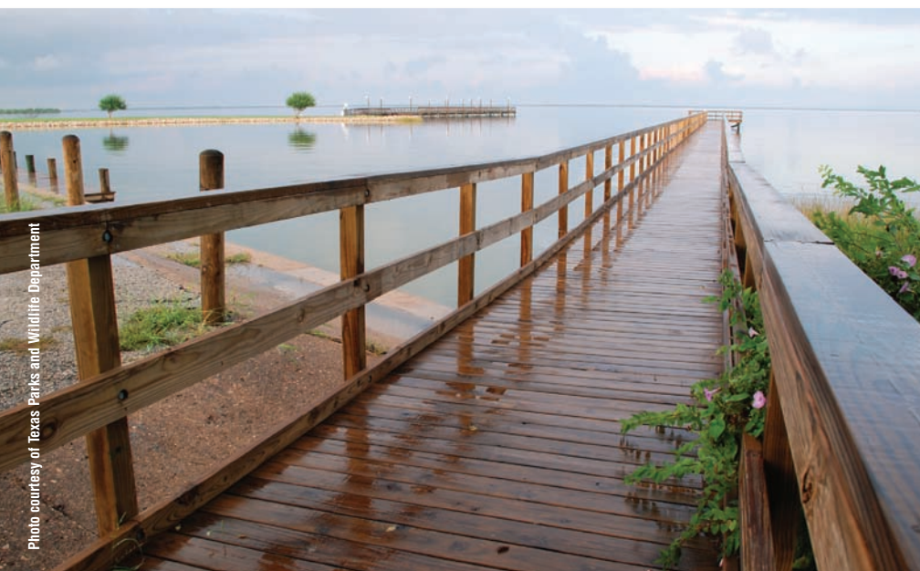
Piers were constructed as part of the restoration project at Lavaca Bay, to offset recreational fishing losses.
