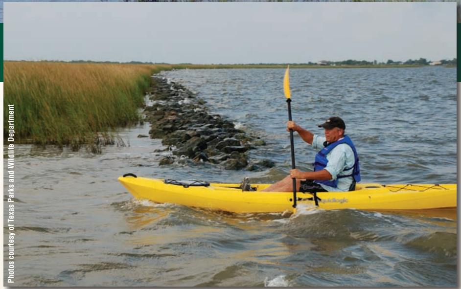
Richard Seiler inspects marsh breakwater at the Lavaca Bay restoration project.
