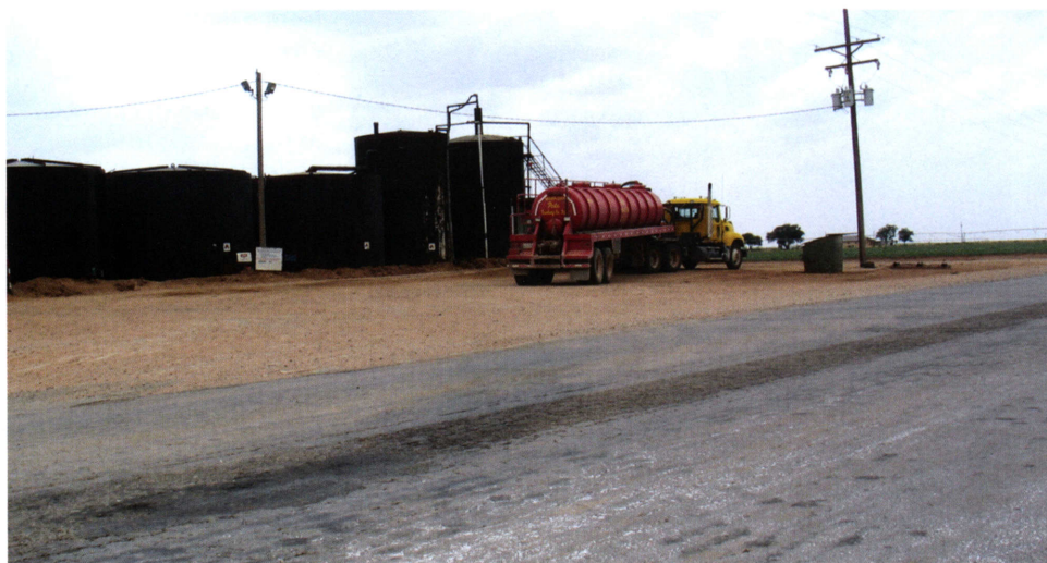
A well fluid station on FM 1585 near Lubbock.
