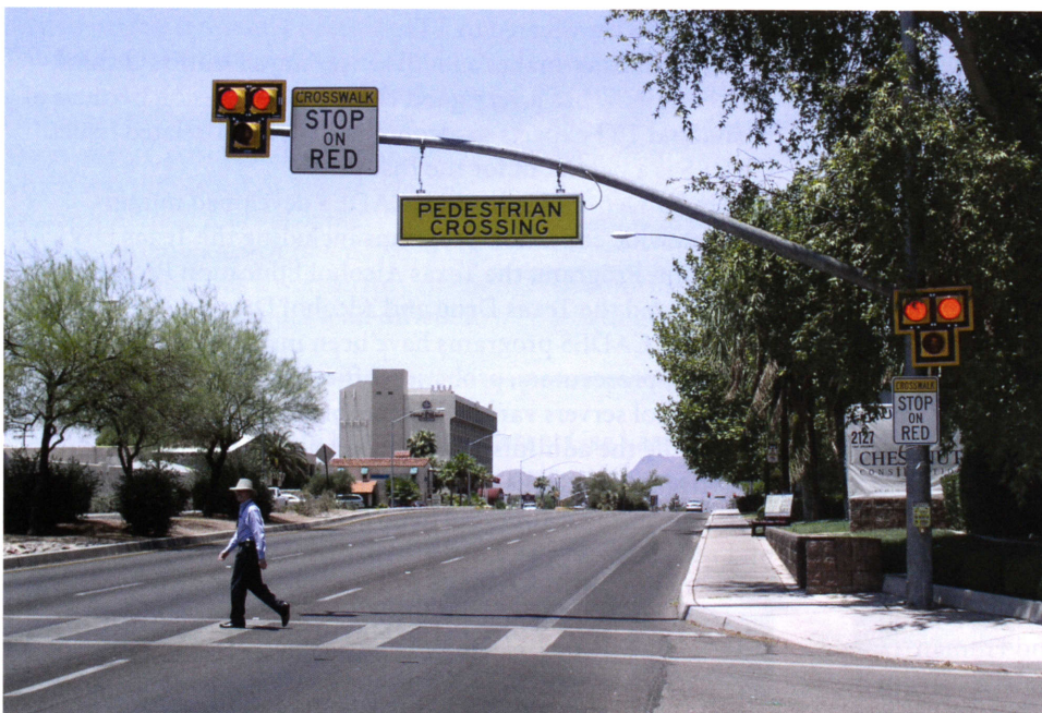
The HAWK treatment was the forerunner of the pedestrian hybrid beacon, which is helping make crosswalks safer for communities across the country.
