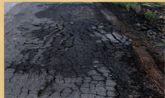
Drainage problems caused by truck traffic are evident on this access road near Abilene.
