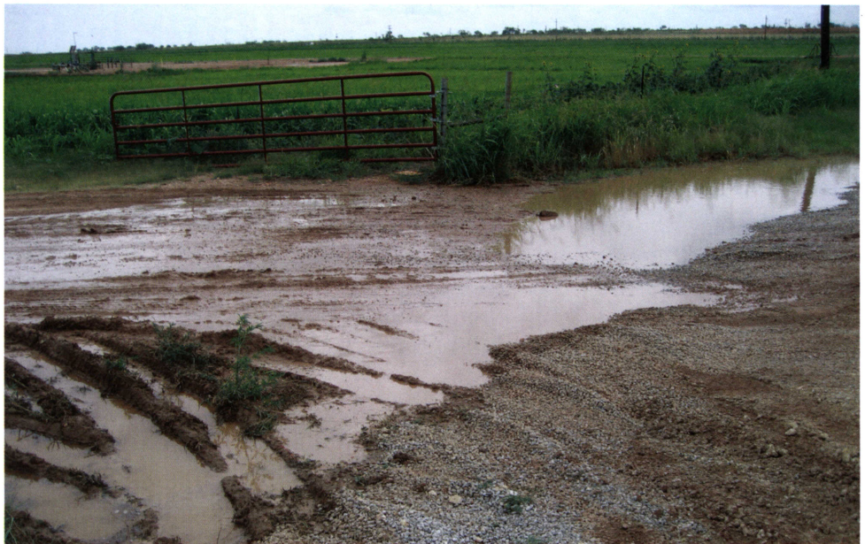
Drainage problems caused by truck traffic are evident on this access road near Abilene.
