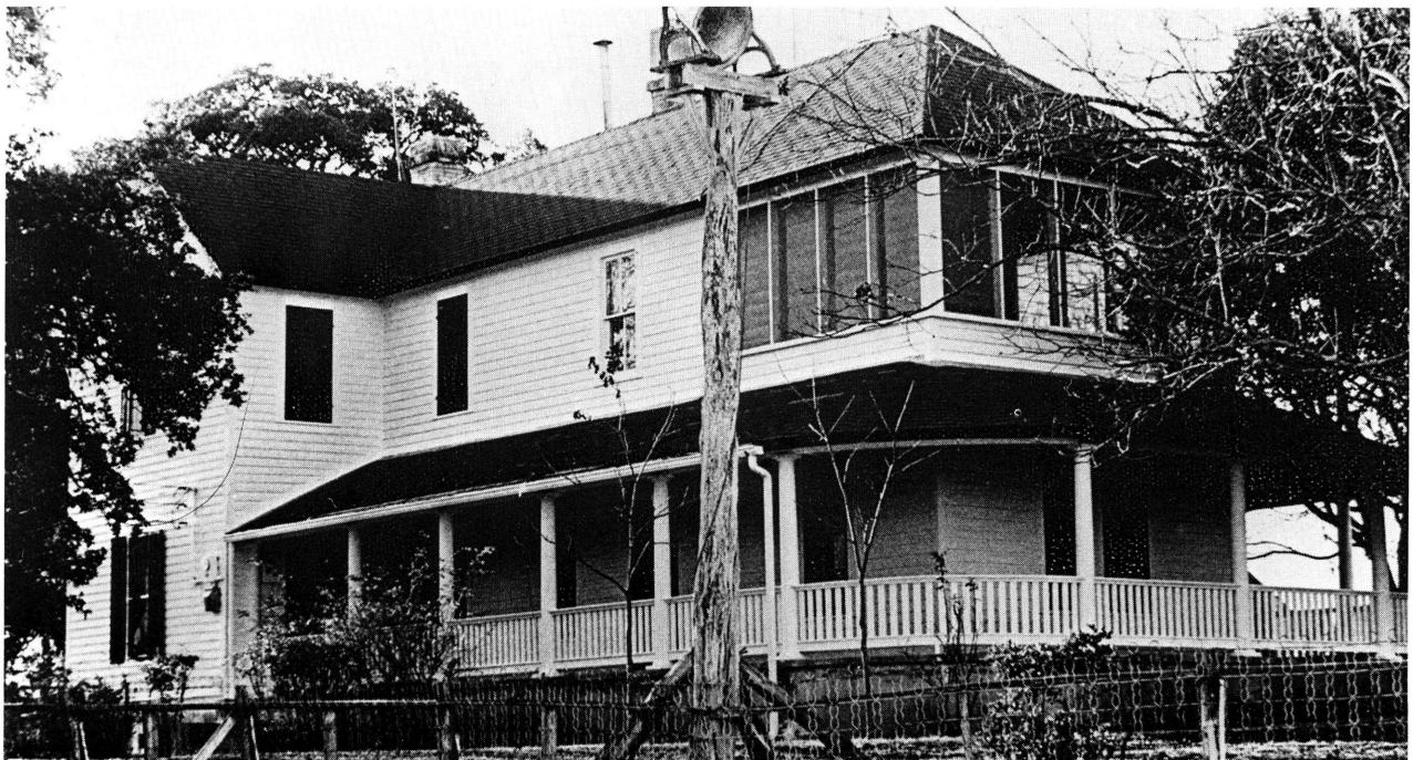
The Real Ranch house is located on Turtle Creek in Kerr County. The home was begun by Founder Caspar Real with additions made by succeeding generations and is maintained by present-owners, Jeanette Boster and Emilie Neill.
