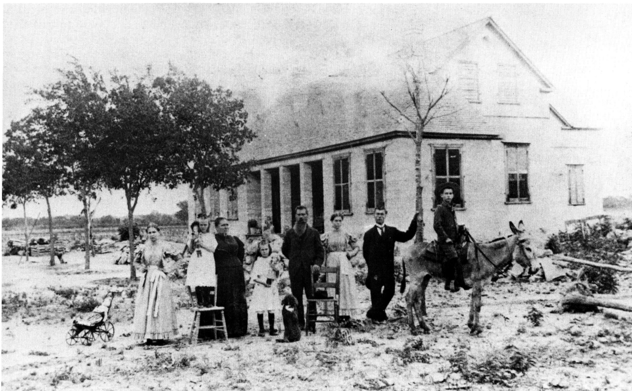
The August Wurzbach family posed for this photograph in 1896 in front of their home on their Menard County farm while it was in the process of construction.
