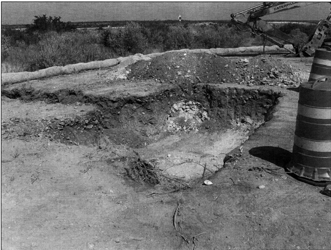
Figure 1.3. Backhoe excavation at previously unknown site 41VV1991, looking northwest.
