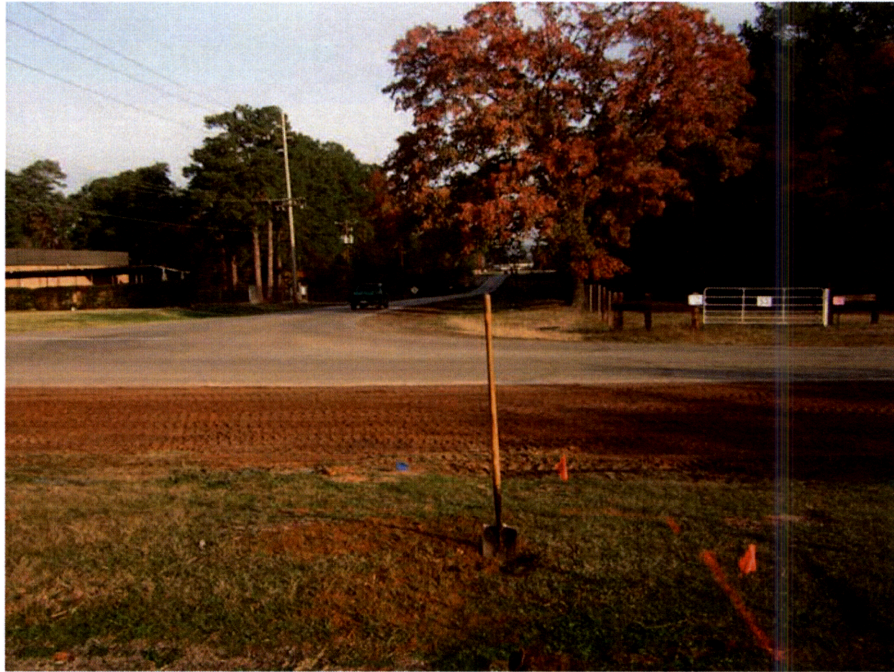
Figure 6 Shovel Test 1 at north end of project at corner of Garland Road and Estes Drive. This is the tie-in for the proposed 12" water line with the existing 16" water line.
