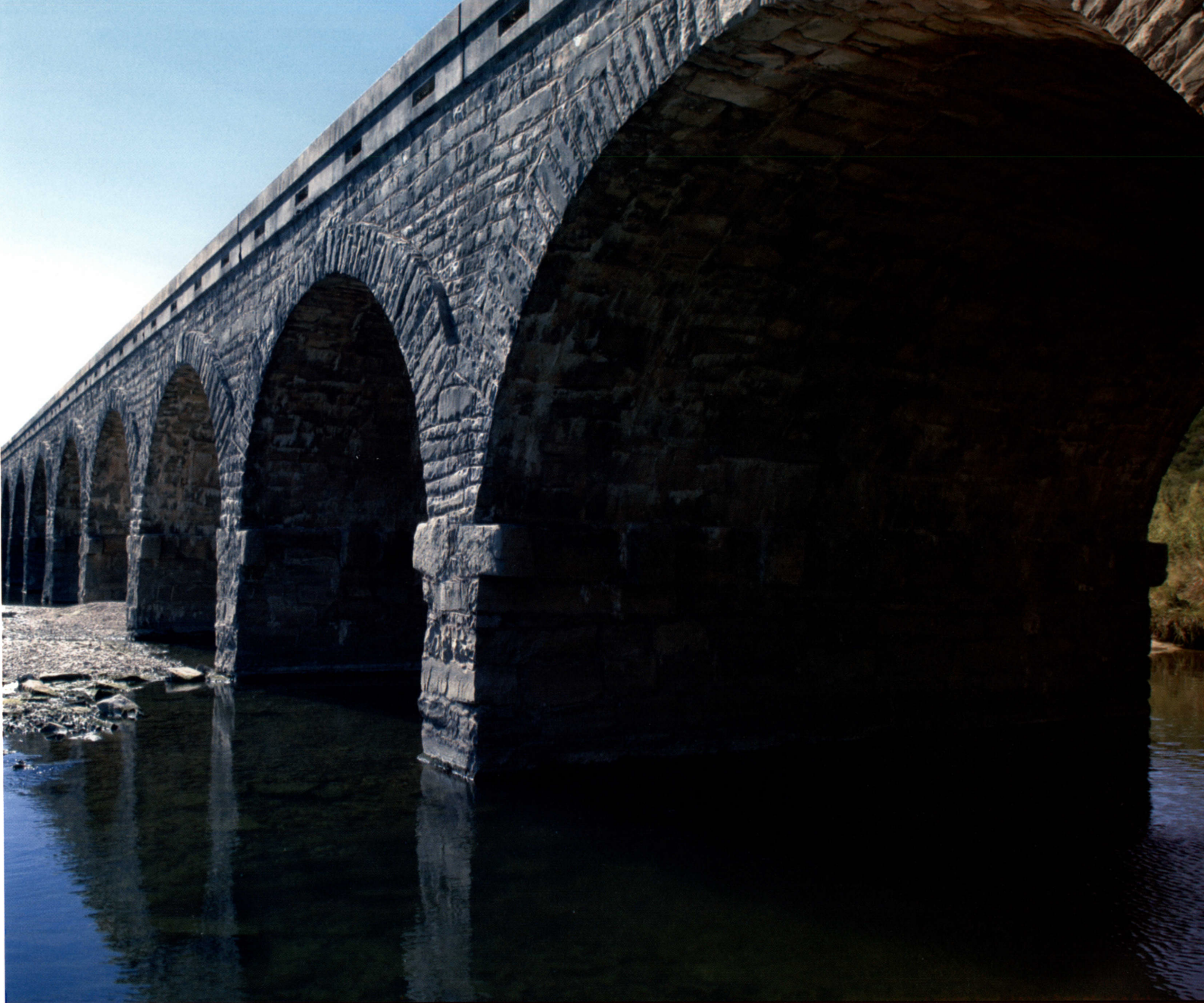
▲ Possum Kingdom Masonry Arch Bridge spans the Brazos River. The 66-year-old bridge is 433 feet long and was designed to withstand floodwaters released from Morris Sheppard Dam upstream. Completed in 1942, it was built of local limestone by WPA workers—many of whom were unemployed coal miners skilled at stonemasonry.
