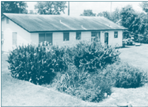
Constructed wetlands are an effective alternative for sewage treatment in some areas where traditional septic systems are impractical.
