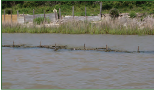
Eroded banks of the GIWW at Mad Island before construction.
