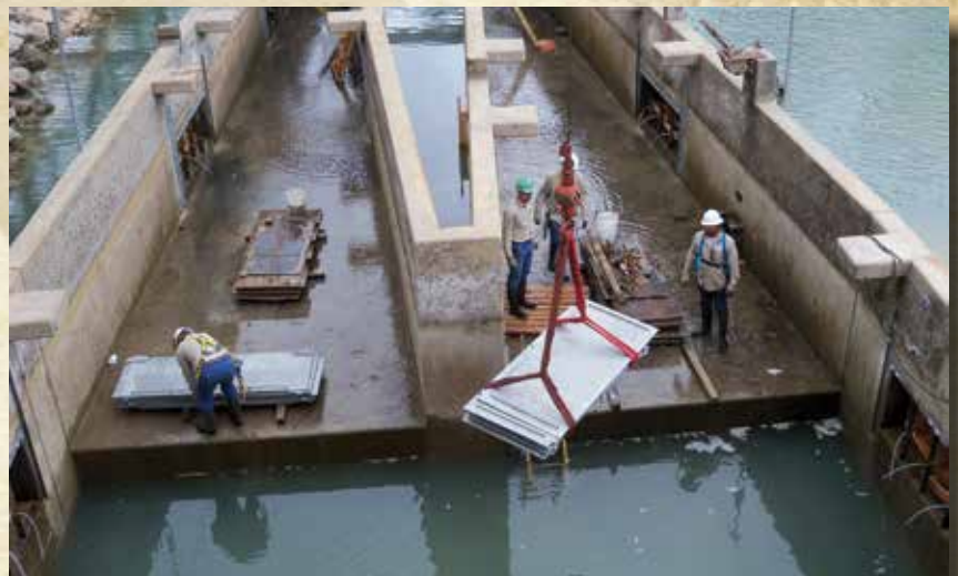
Weir Repair Work
