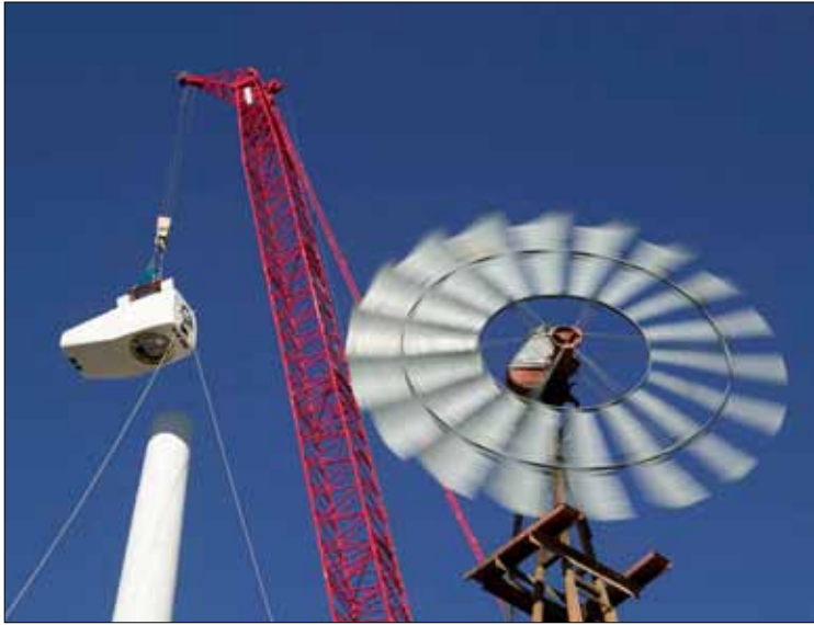
Wind Farm Construction
