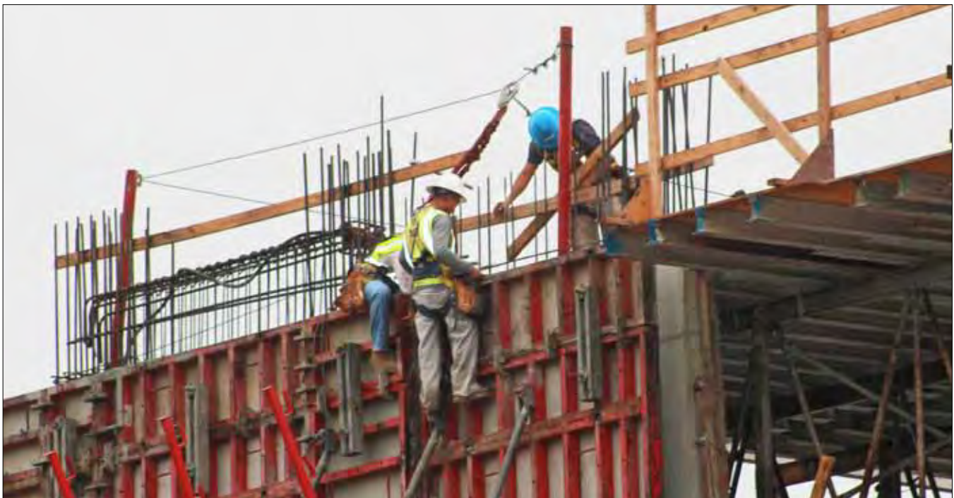
Construction Work in Downtown Austin PHOTO: Courtesy of Ginger Lowry
