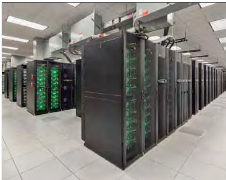
"Stampede" Supercomputer at the Texas Advanced Computing Center, The University of Texas at Austin PHOTO: Courtesy of Texas Advanced Computing Center
