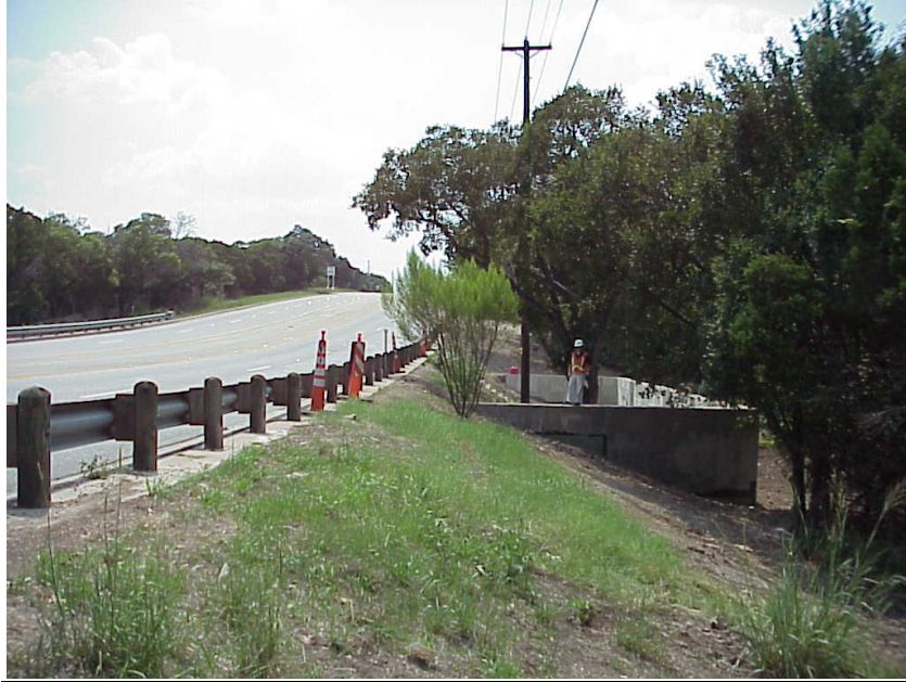
Figure 4.1. Entrance Weir Culvert Structure to Mimic Overtopping of Pre-Improved Roadway.
