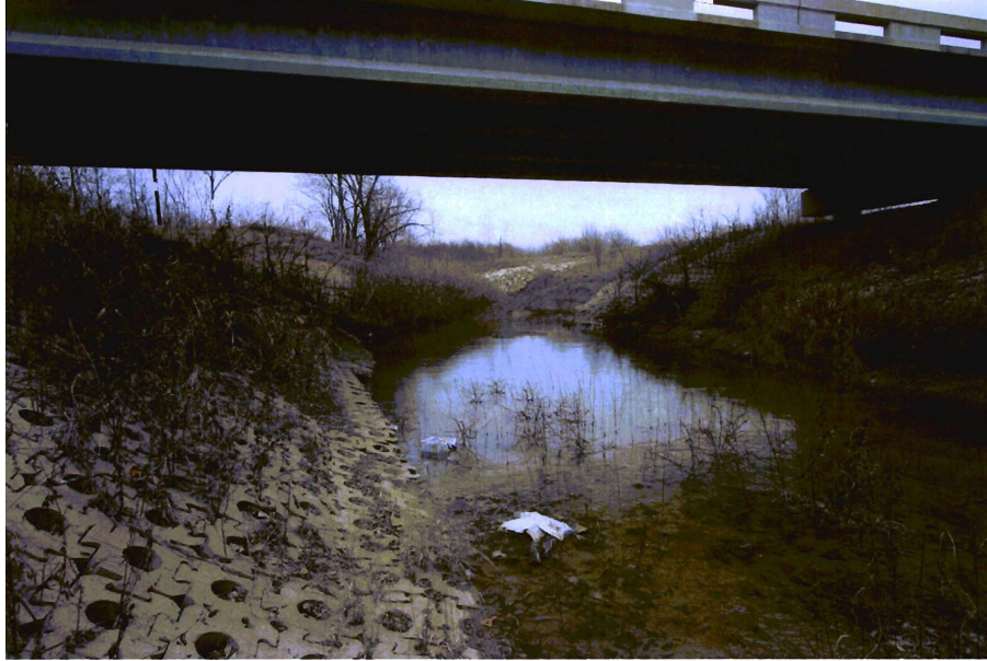
Figure 4.6. Articulating Concrete Blocks Stabilize the Channel Slopes of the North Sulfur River, while Permitting Infiltration and Vegetation.
