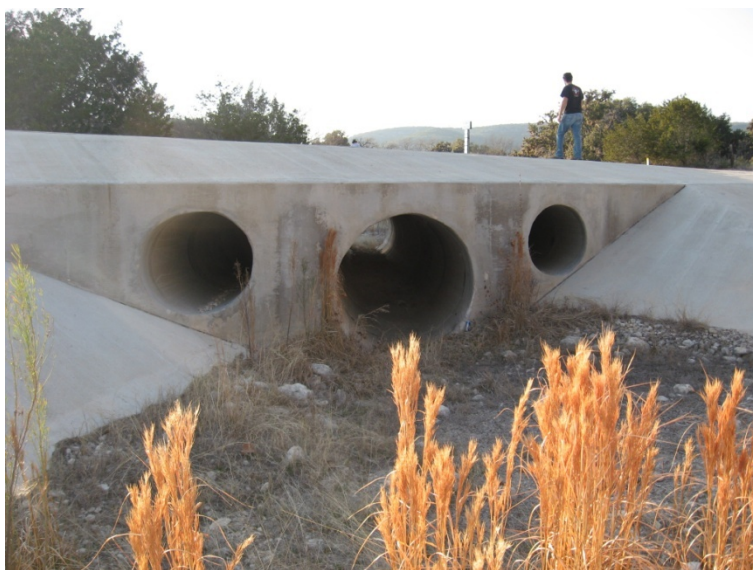
Figure 4.5. The Upstream Side of the Same Site Shown in Figure 4.4, but with a Staggered Barrel Culvert System Having Been Installed for Two Years.
