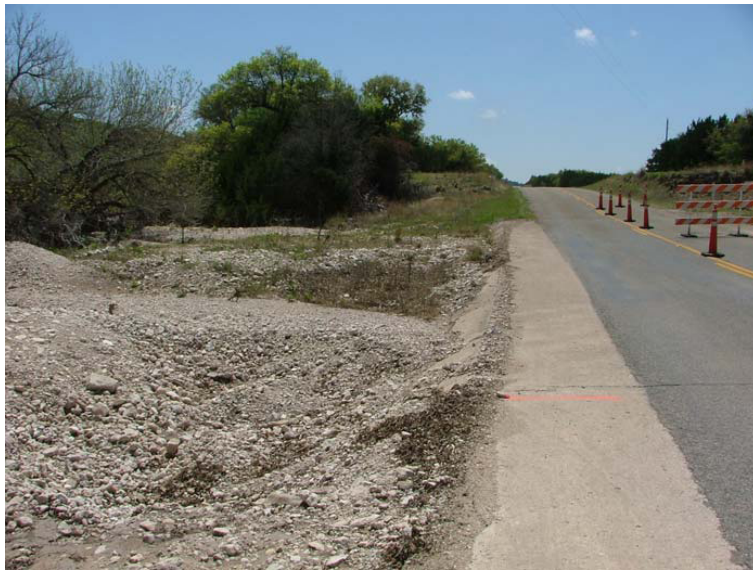
Figure 4.4. The Upstream Side of a Traditional Vertical Sag/Culvert Crossing with Accumulated Bed Load Material (Herrmann, 2007).
