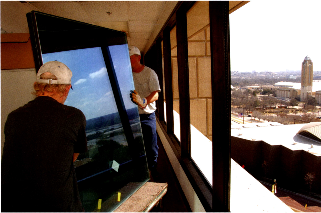
Workers install more energy efficient windows in the Education and Administration Building.
