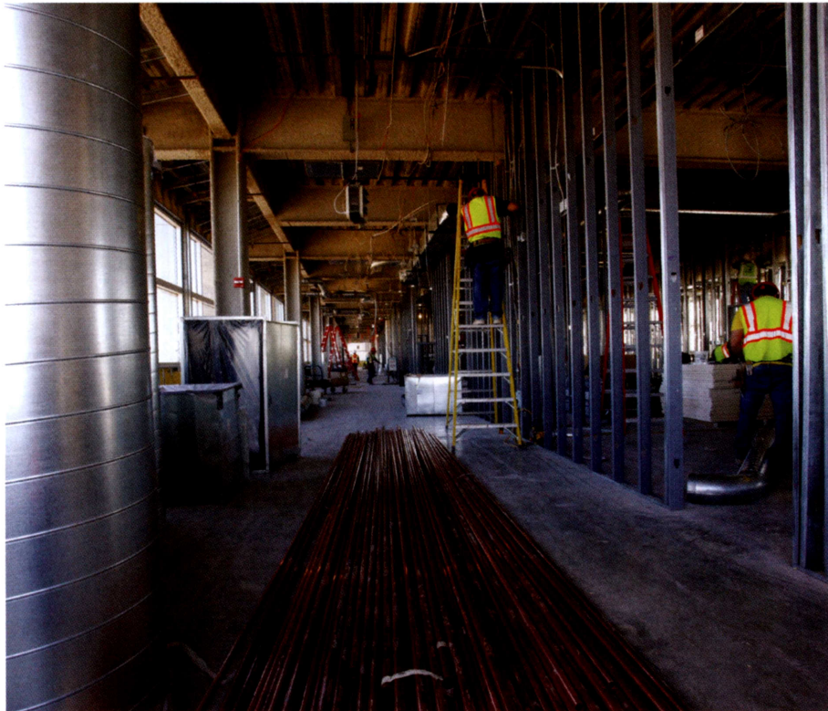
Work is progressing in the MET Building.
