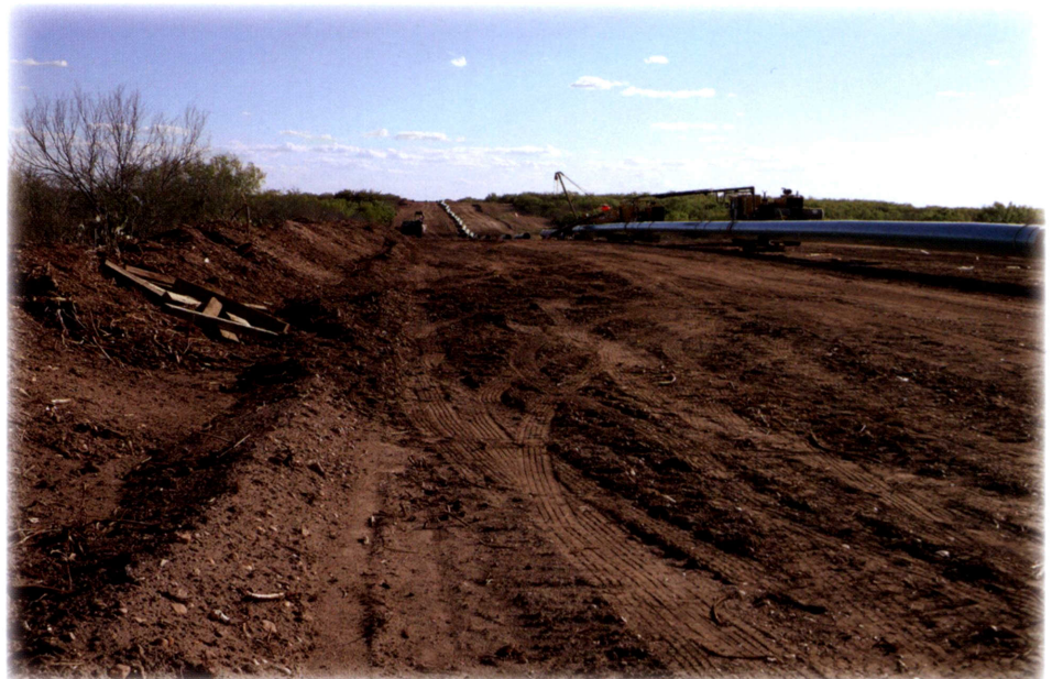
Eagle Ford Shale pipeline installation.
