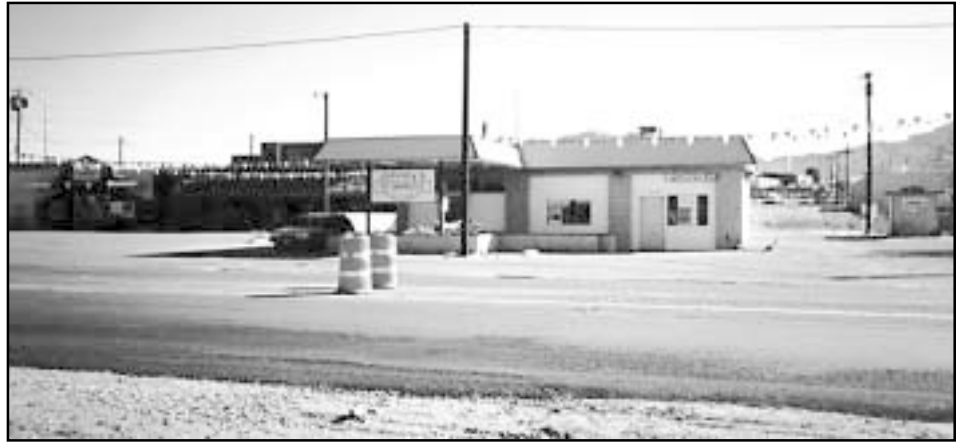
What is now a barbecue restaurant was formerly a service station and turned out to have sub-surface contamination from buried petroleum storage tanks.
