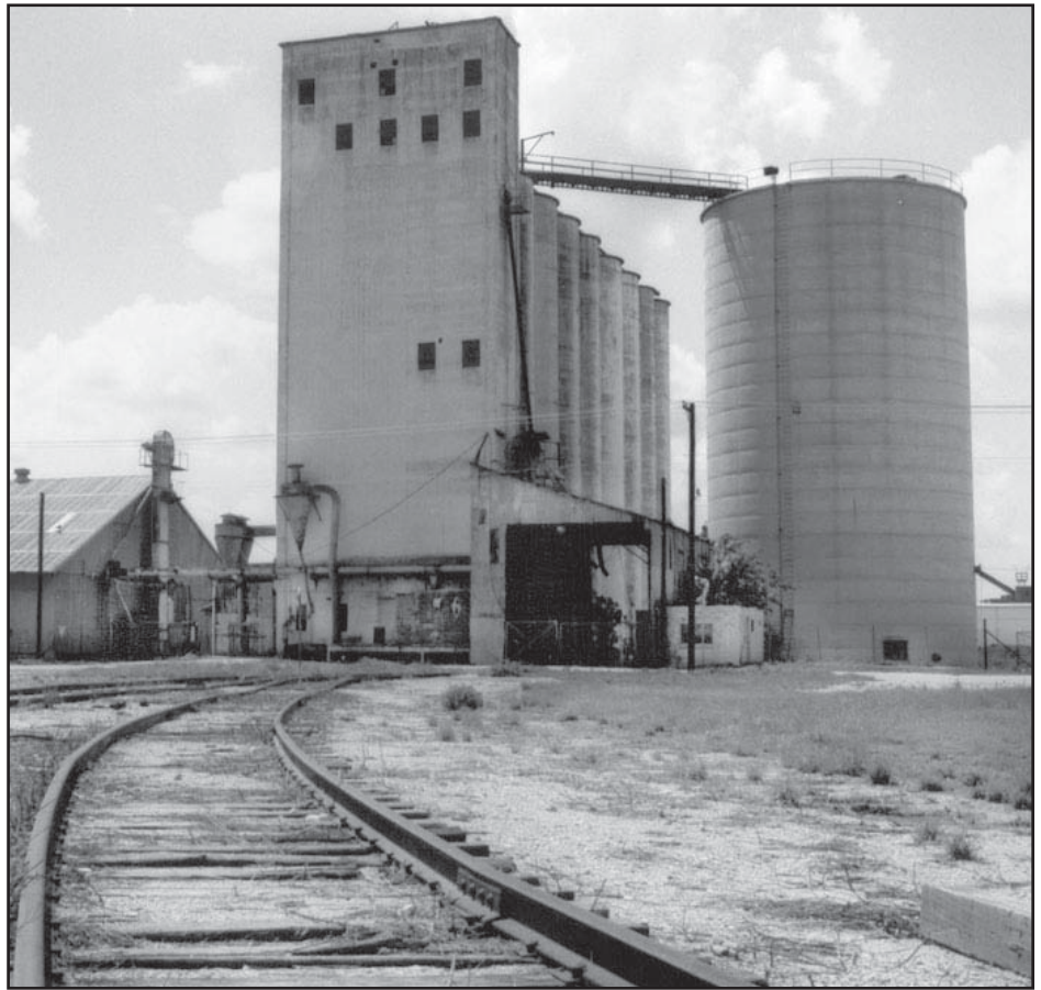
Continental Grain Elevator and Warehouse in downtown Brownwood.
