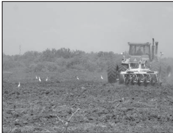
Work continues on mitigation project.
