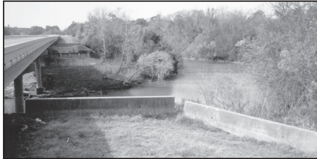
The old bridge approach, where concrete remains, was abandoned in favor of a higher elevation approach 30 feet over. (Houston District photo)
