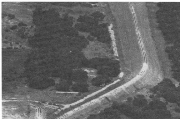
Salado Site 12 Floodwater retention dam
