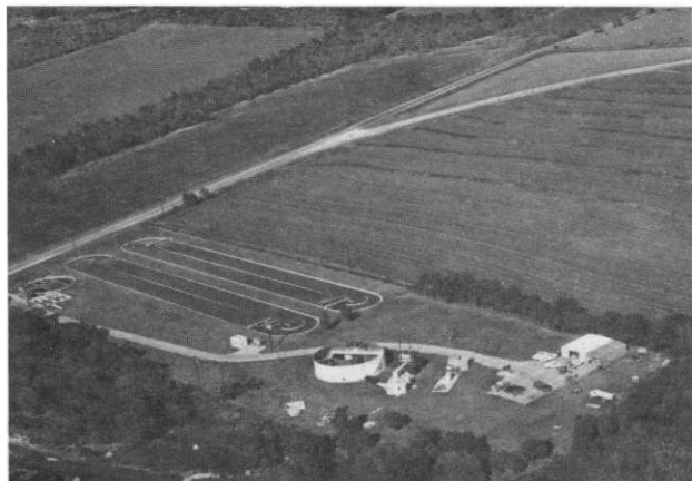
Salatrillo Sewage Treatment Facility, Bexar County.
