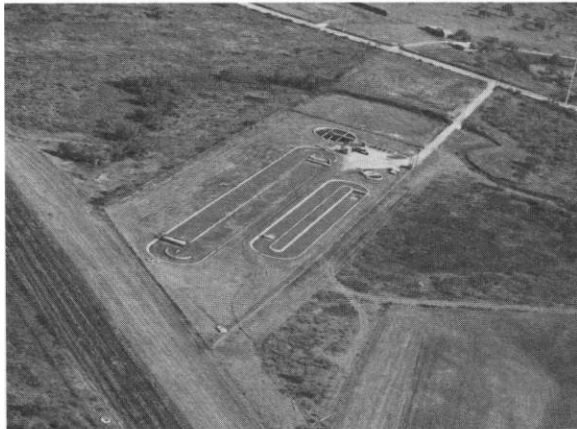
Martinez Sewage Treatment Facility, Bexar County.
