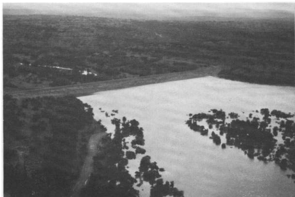
Salado Site 8 Retaining floodwater
