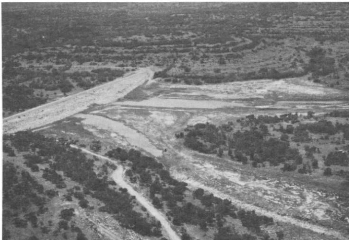
Salado Site 8 Floodwater retention dam
