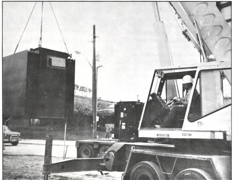
Heavy Hauling Crew members Little (left) and Bermea (right) guide transformers in one of the River Center vaults.
