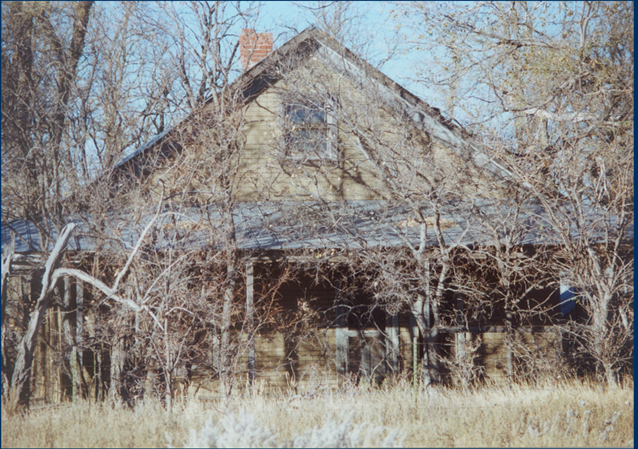
South side of Moore house prior to salvage
