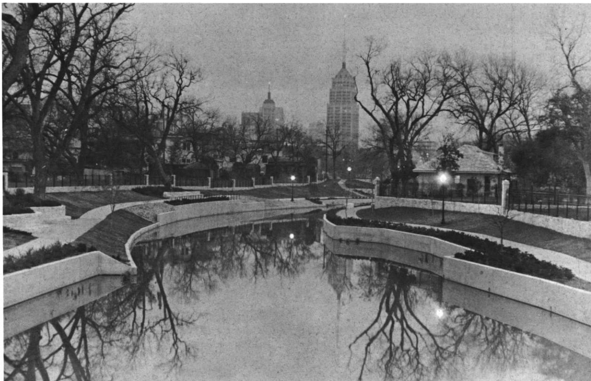
Winter scene of the San Antonio Channel Improvements project, South Alamo to Arsenal Street.
