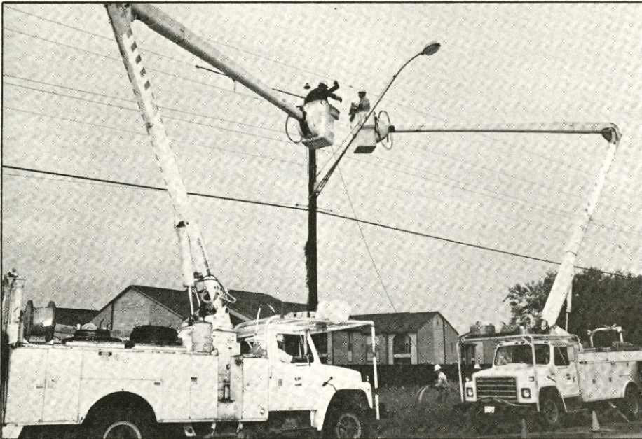
Linemen correct one of 67 electric circuits affected by the unexpected rainstorm.
