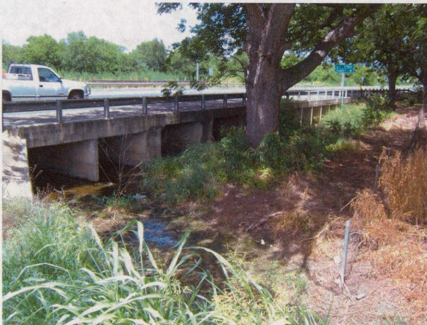
Figure 2.0 – Parkers Tributary at Hwy 90 Eastbound
