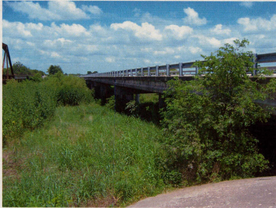
Figure 1.0 – Seco Creek at Hwy 90 Westbound
