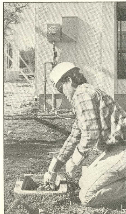
CPS gas serviceman connects gas service.
