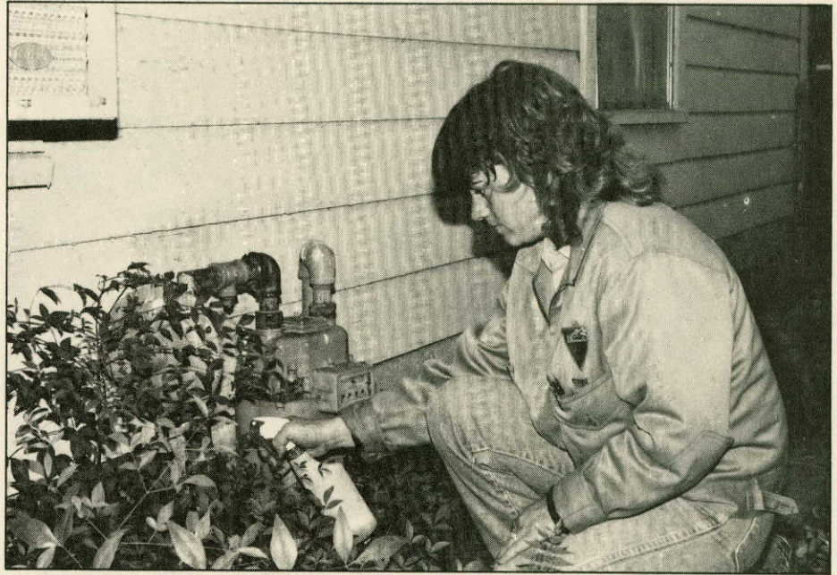
Gas Operations Trainee Martha Carnes checks a CPS meter for gas leaks.
