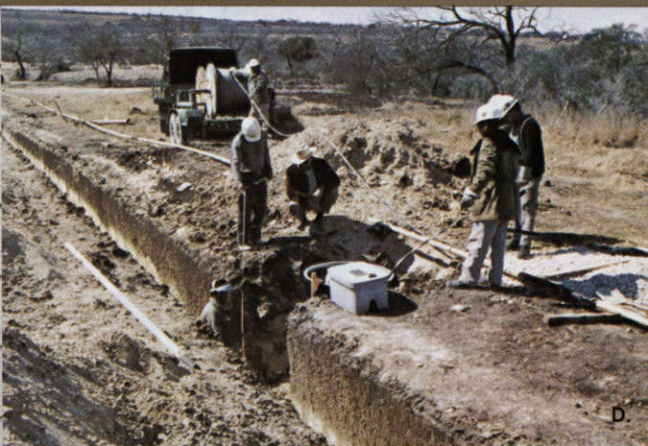
A. Sommers Unit No. 1, rated at 430 MW, will be on line in the spring. B. Job conference on the scene. C. Skilled professionals serve customers. D. Joint trenching with URD cable under gas pipe. E. Radio dispatching insures prompt service.
