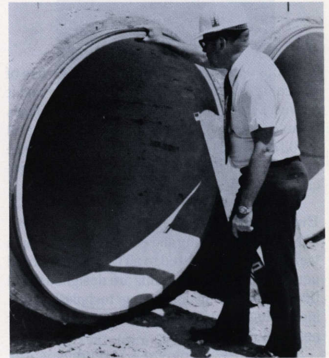
City Water Board safety inspector examining 60-inch pipe before installation.
