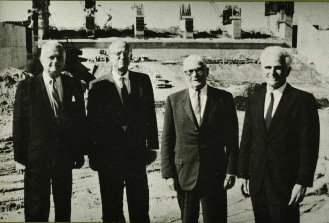
Four members of the Board of Trustees (above) are pictured on a tour of the CPSB's Calaveras power plant and dam project. Left to right are: J. H. Morse, Albert Steves III, John R. Locke and Leroy G. Denman, Jr. In other picture, Mayor W. W. McAllister, left, ex-officio member of the Board of Trustees, reviews computer operations with O. W. Sommers, General Manager.
