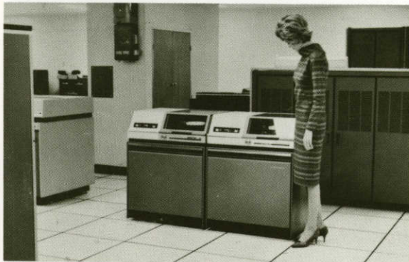
Random access disc drives store 5,000,000 bits of data.
