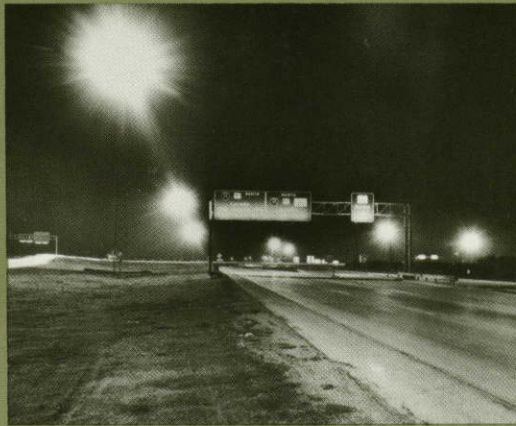
New 100-ft. towers at expressway interchanges feature clusters of ten 55,000 lumen fixtures.
