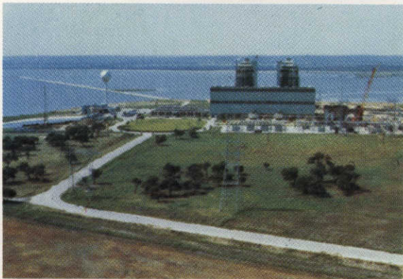
A third generating unit, of 417,000 kw capability, is being added at the Braunig power plant.
