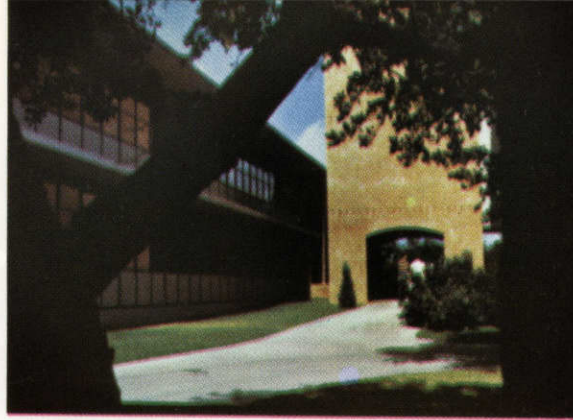
Entranceway to new Engineering Science Building, Trinity University
