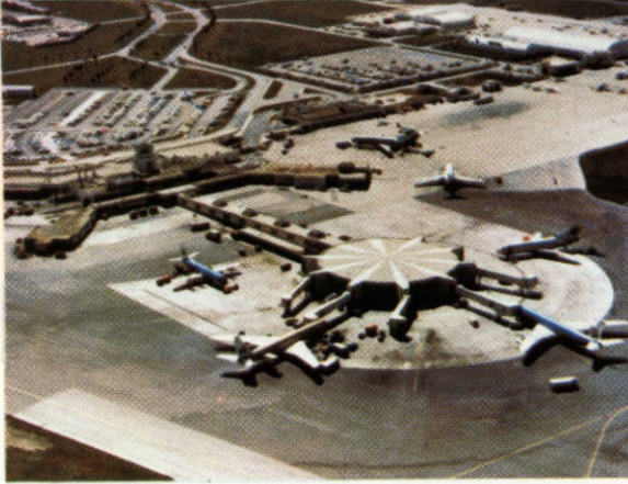
International Airport with direct jet service throughout the Western Hemisphere
