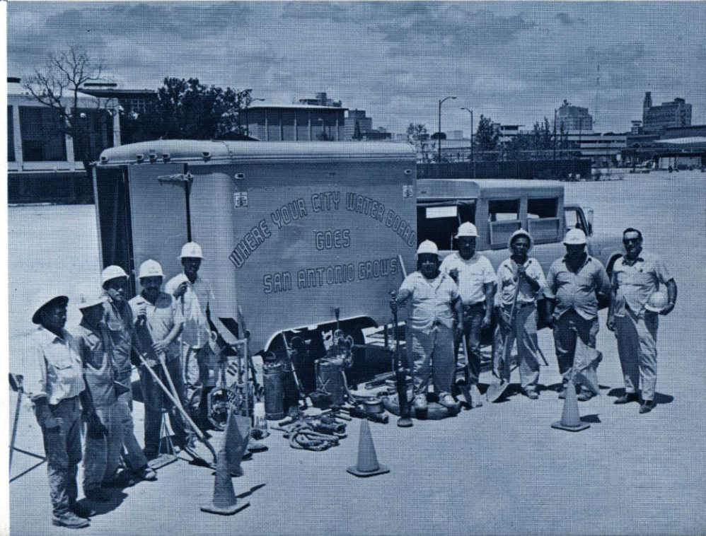
(Right) This 10-foot tool trailer pulled by a \frac{3}{4} -ton truck is one type of mobile unit used on main construction projects. This 10-man crew displays a variety of the tools and safety equipment used on construction projects.
