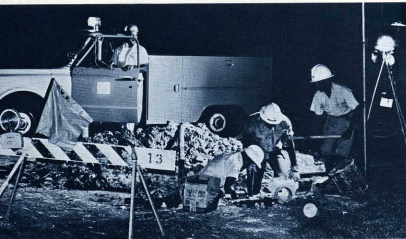
(Lower, center) A 20-inch gate valve is salvaged in an urban renewal area project. The pneumatic metal saw moves on a chain around the large main as it saws through the thick pipe. This gate valve will be reconditioned and then reused in the water distribution system.
