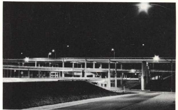
Brightly lighted expressways reduce accidents.
