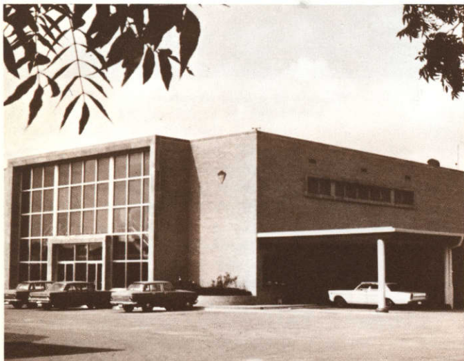
Gas distribution building houses engineers, technicians and service facilities.
