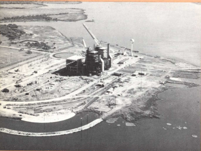
Cooling water is drawn from lake through underground pipes and discharged after condensing the steam.
