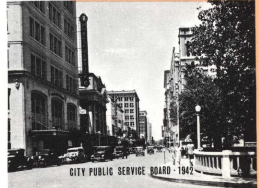
Former CPSB main office on St. Mary's Street.
