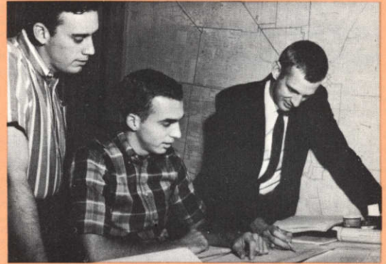
Loading of downtown underground distribution network is frequently checked.
