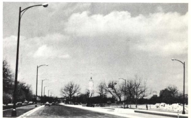
Approaches to HemisFair served underground.
