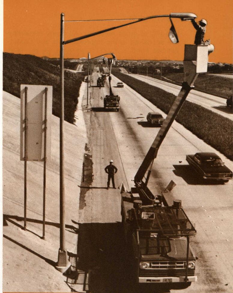
Street light installations included 173 expressway, 715 arterial and 456 residential lights, making San Antonio with a total of 28,935 installed, one of America's best lighted cities.
