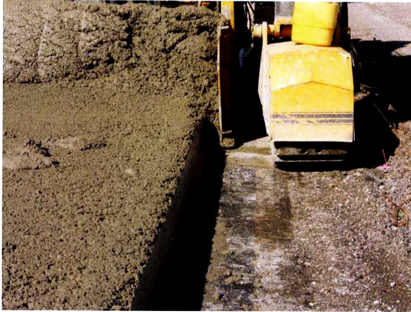
Figure 10. Envelope Outside Edges of Bottom Lifts (Adopted from Gillen and Vavrik 2012).
