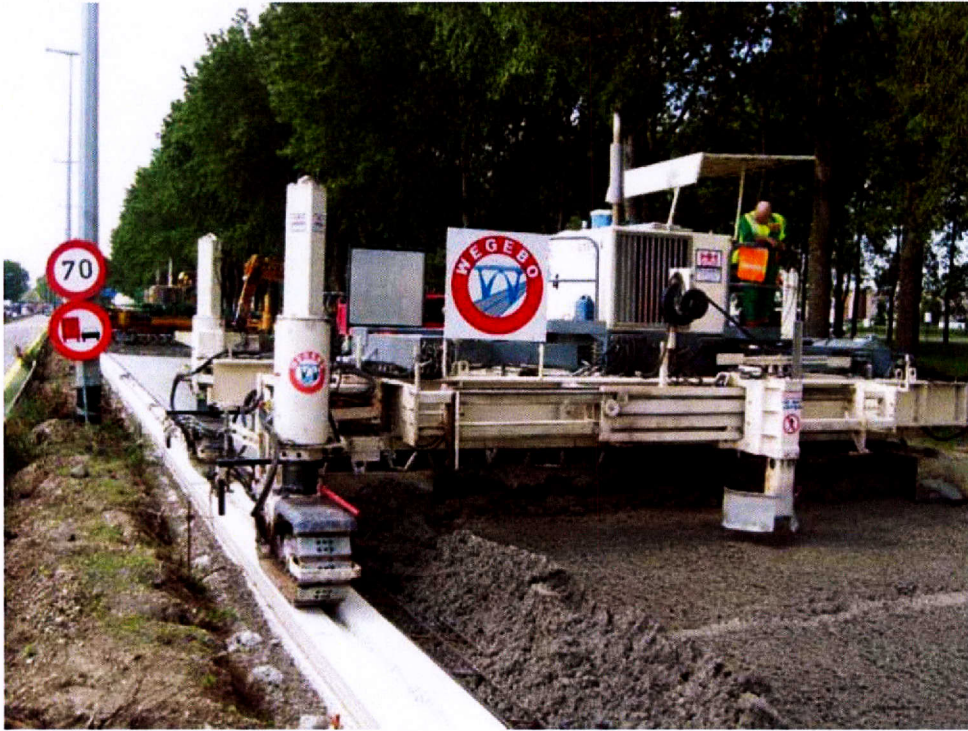
Figure 19. CRCP Construction in E34 Motorway Construction (Ren 2008).
