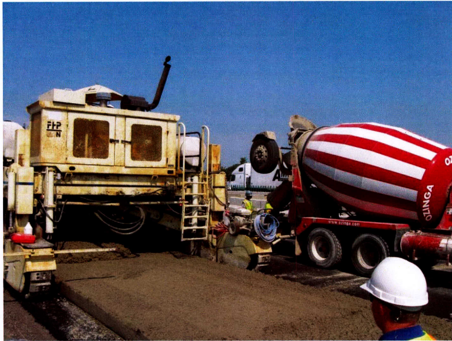
Figure 23. 2LCP Construction in Illinois Tollway (Photo Courtesy of Meininger).
