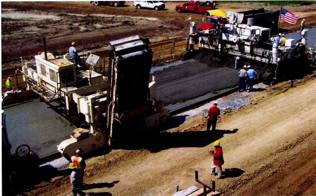
Figure 20. 2LCP construction in Kansas I-70 Project (Gerhardt 2013).
