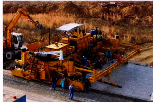
(b) 2LCP with single paver for 2LCP implement (Gomaco 2012)
