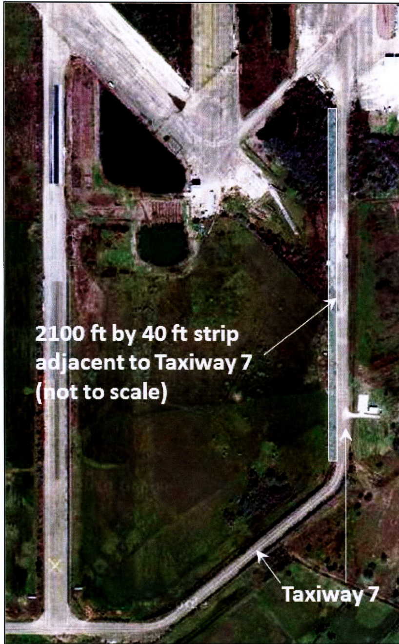
Figure 3. Approved Site along Taxiway 7 for Construction of New Test Tracks.
