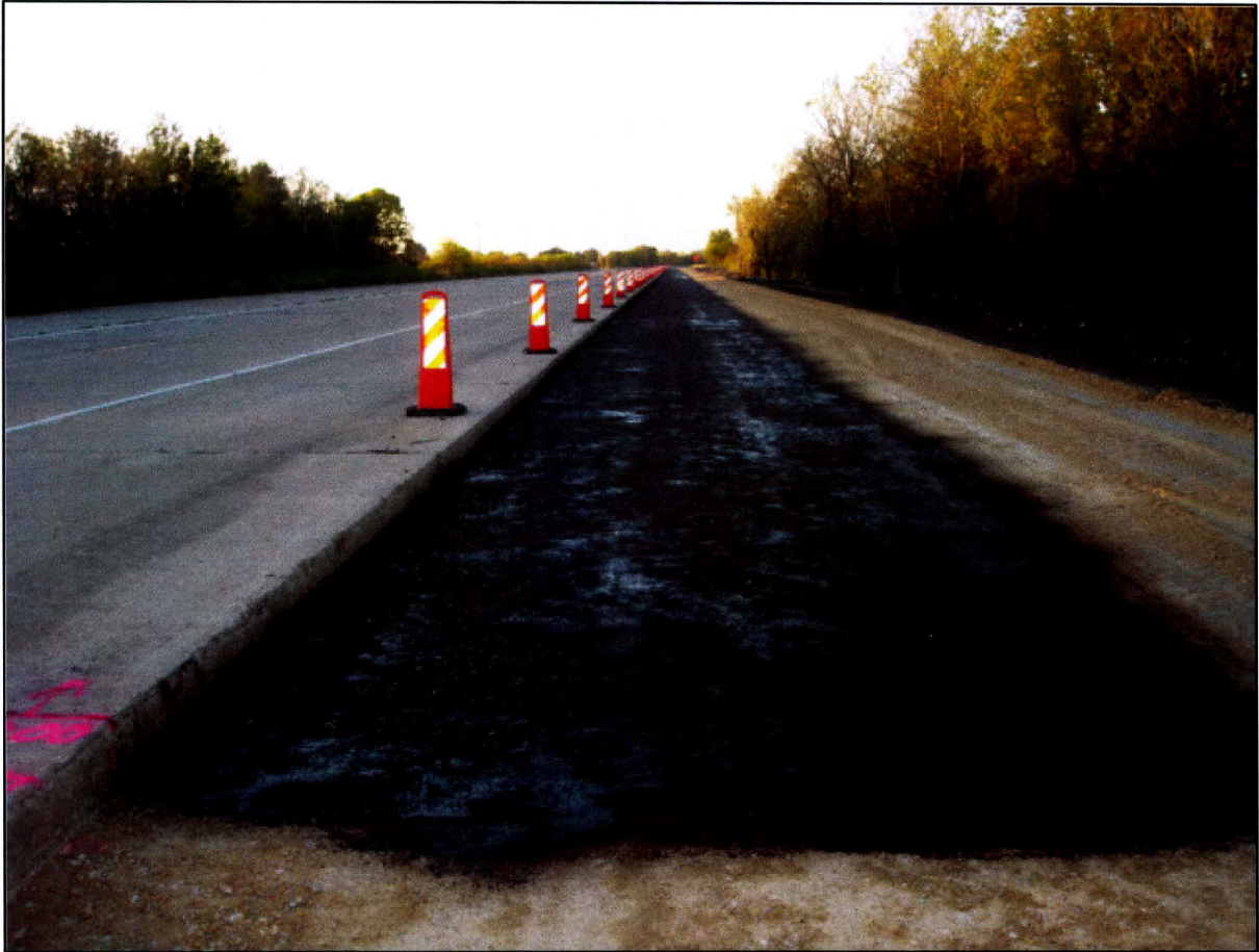
Figure 30. Tack Coat Applied to Flexible Base.
