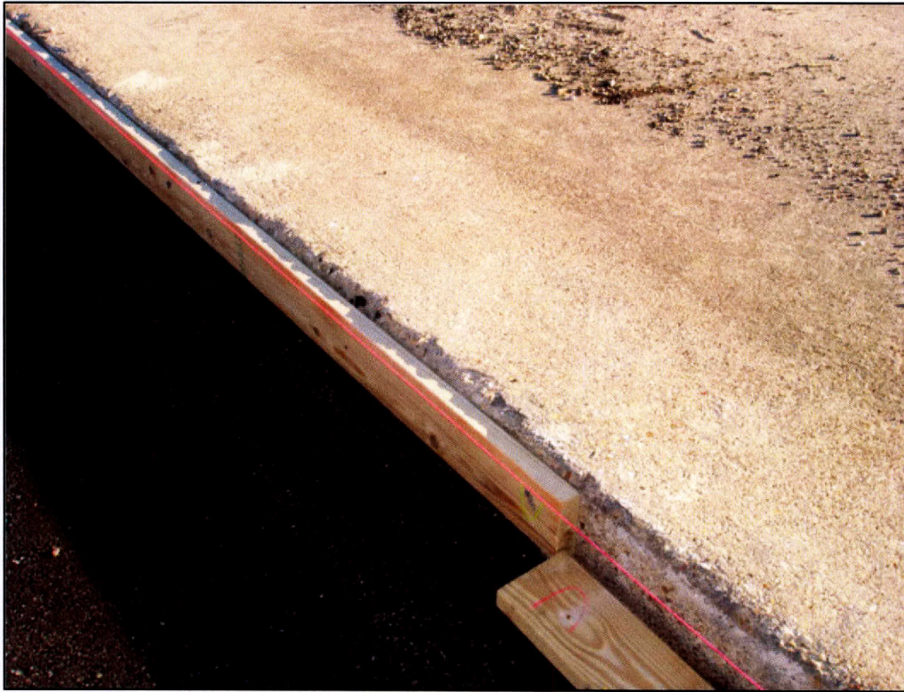
Figure 35. Placement of Form along East Side of Type C Base.
