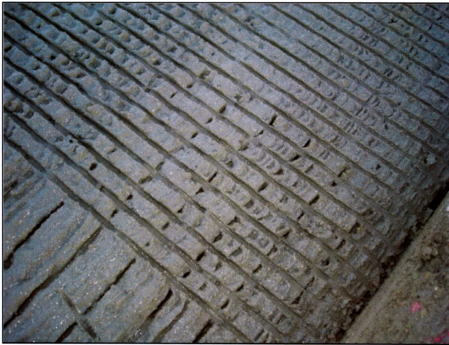
Figure 40. Change from Longitudinal Tines to ½-inch Transverse Tines.
