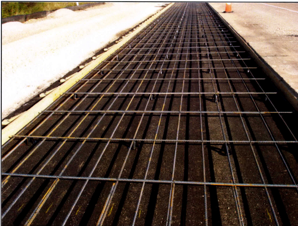
Figure 36. Reinforcement Placed for CRCP Test Track.
