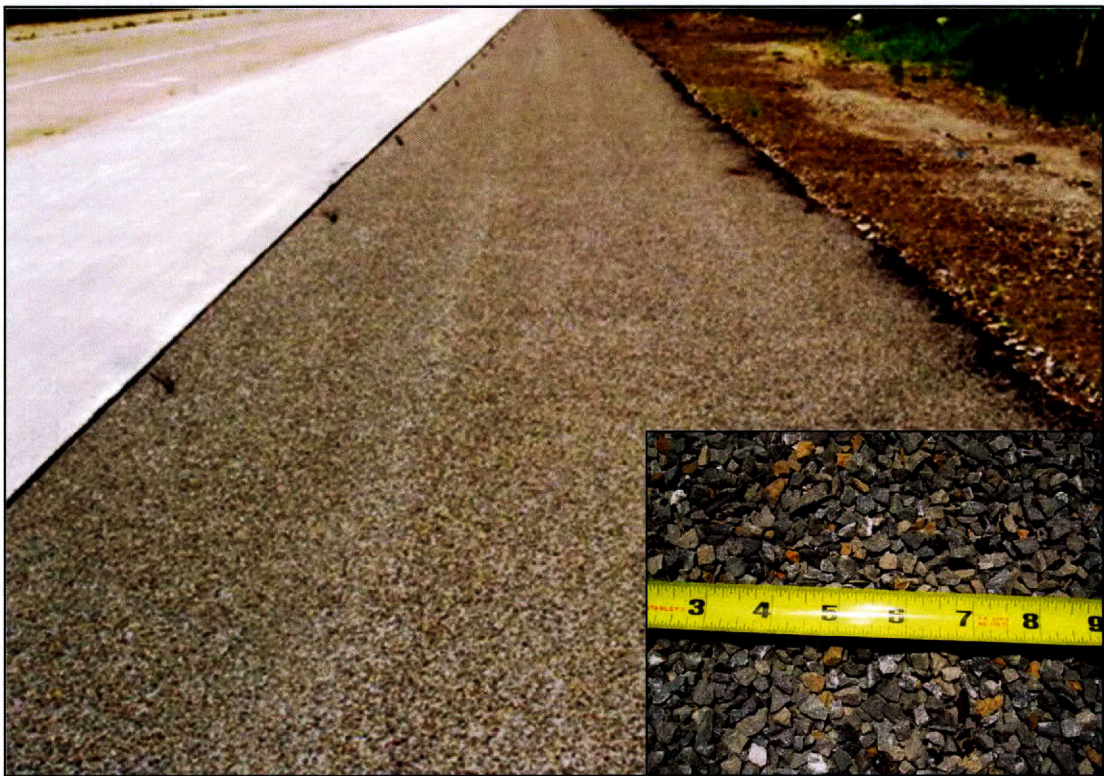
Figure 55. Inverted Prime Section.
