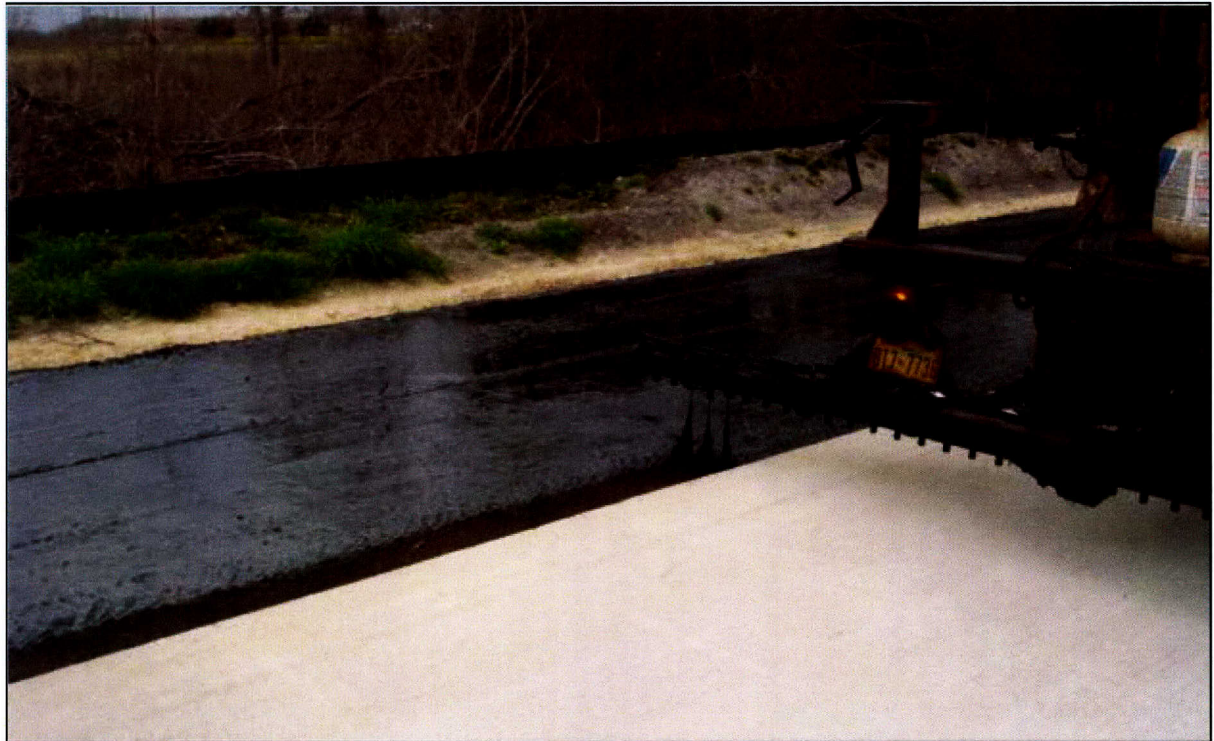
Figure 45. Finishing Asphalt Application on Flexible Base for Surface Treatment.
