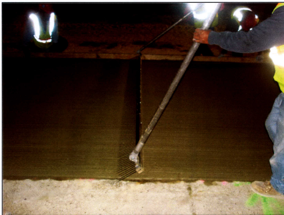
Figure 39. Concrete Surface Textured with Longitudinal Tines.
