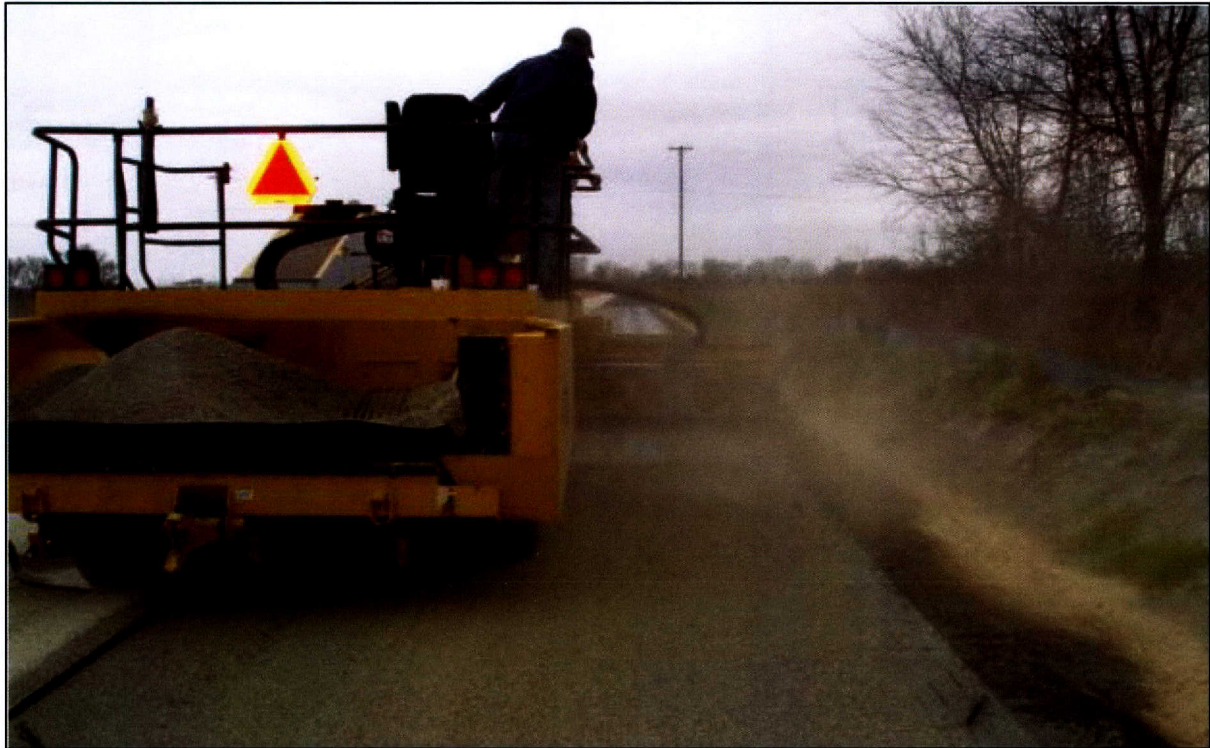
Figure 47. Chip Spreader Applying Grade 5 on Outside Half of Inverted Prime Section.
