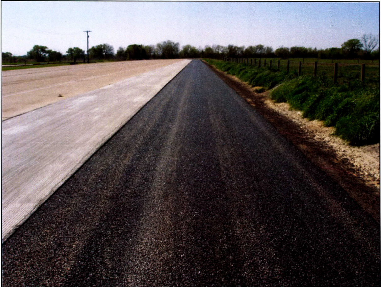
Figure 49. PFC Section Adjacent to Longitudinally Tined CRCP Section.
