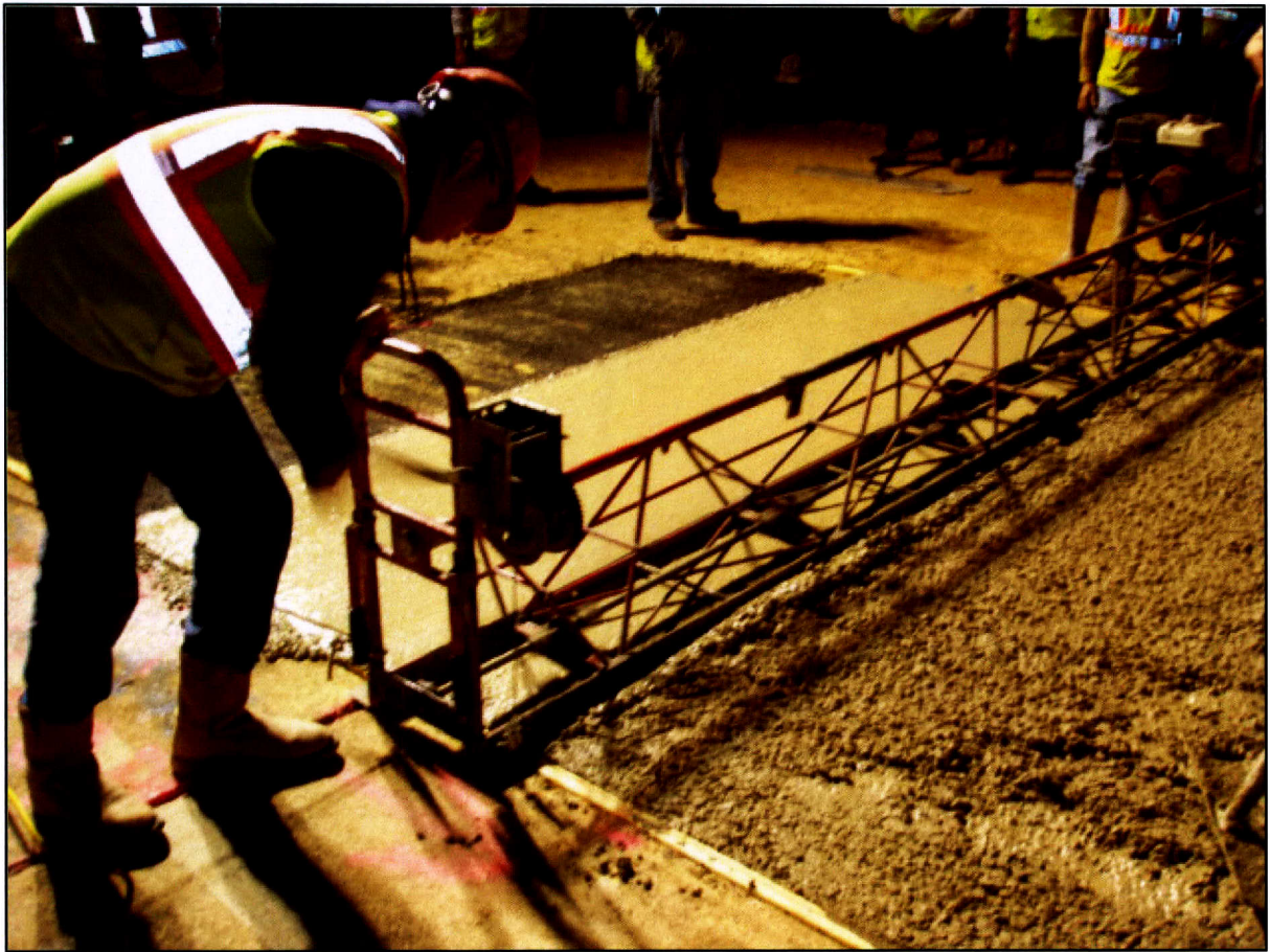
Figure 37. Vibrating Screed Used to Place the Concrete Mix.
