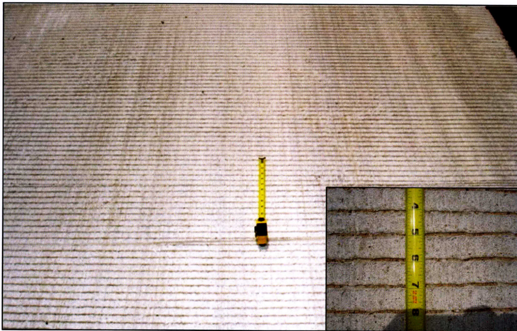
Figure 53. One-inch Transversely Tined CRCP Section.
