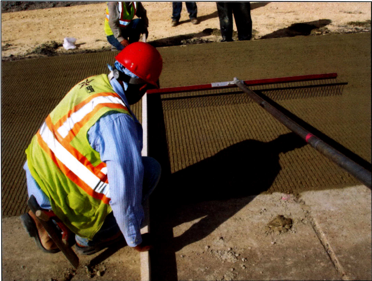
Figure 42. Concrete Surface Texture with 1-inch Transverse Tines.
