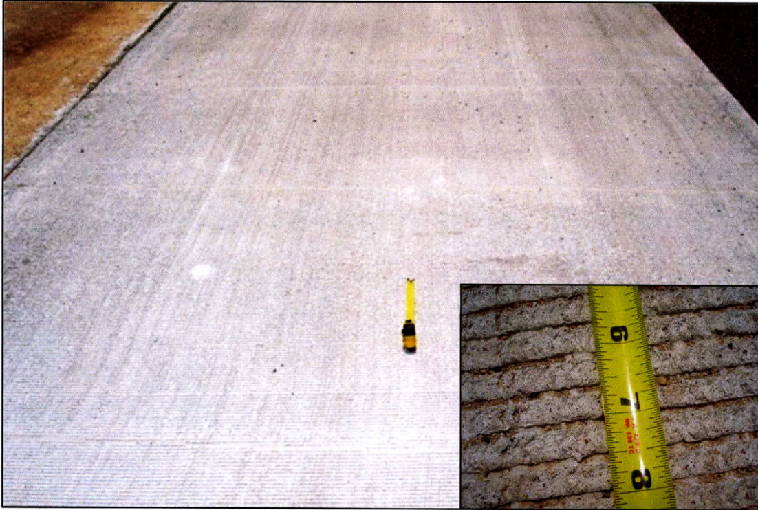
Figure 52. Half-inch Transversely Tined CRCP Section.
