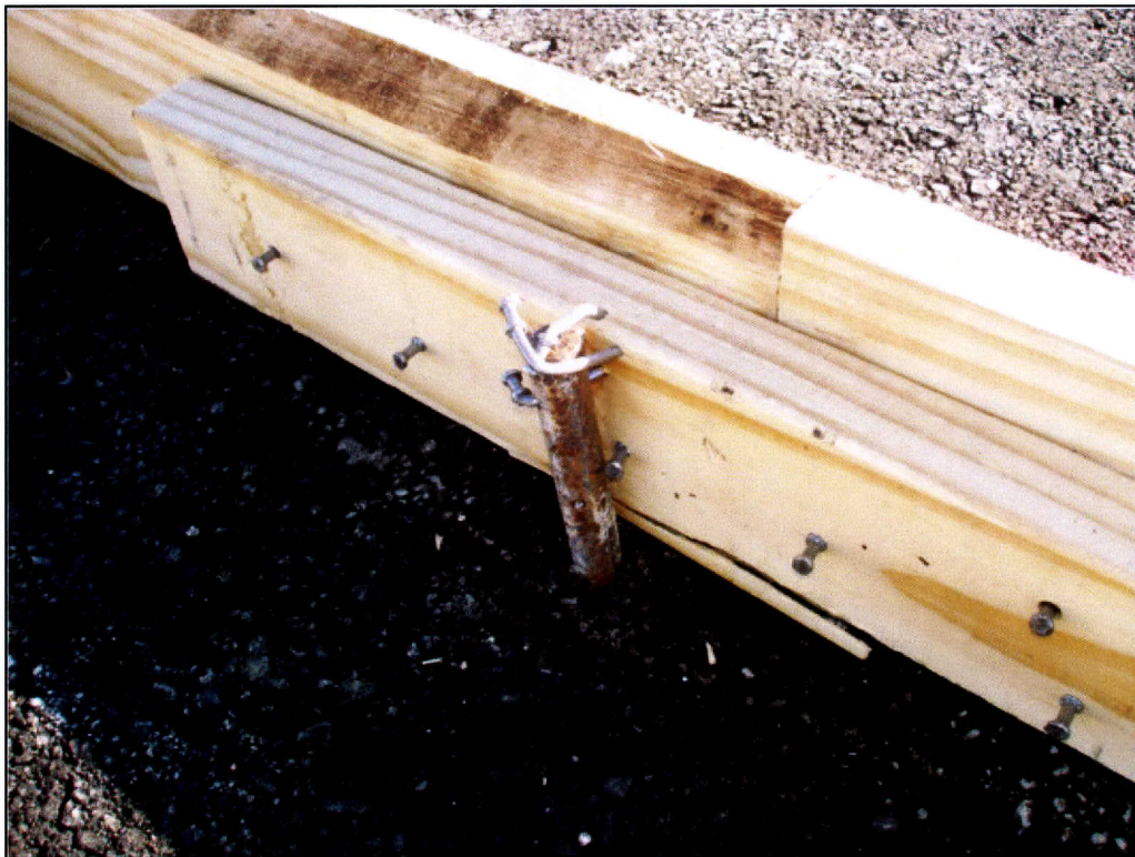
Figure 34. Joint between Form Segments on West Side of Type C Base.
