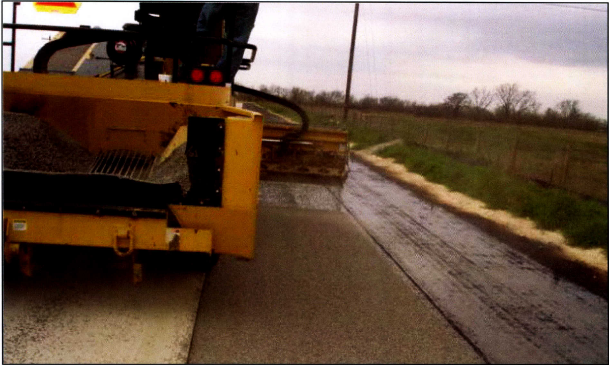
Figure 46. Chip Spreader Applying Grade 5 on Inside Half of Inverted Prime Section.
