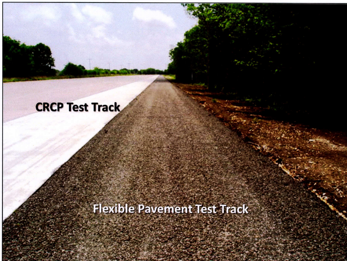
Figure 50. New Test Tracks for Profiler Certifications.
