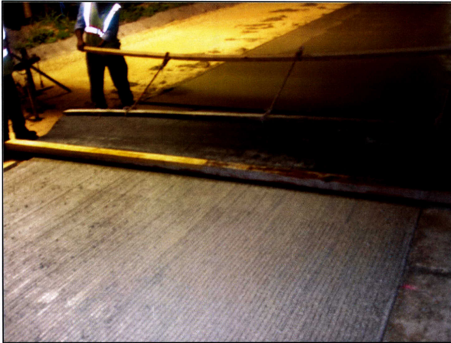
Figure 38. Concrete Surface Textured with Carpet Drag.
