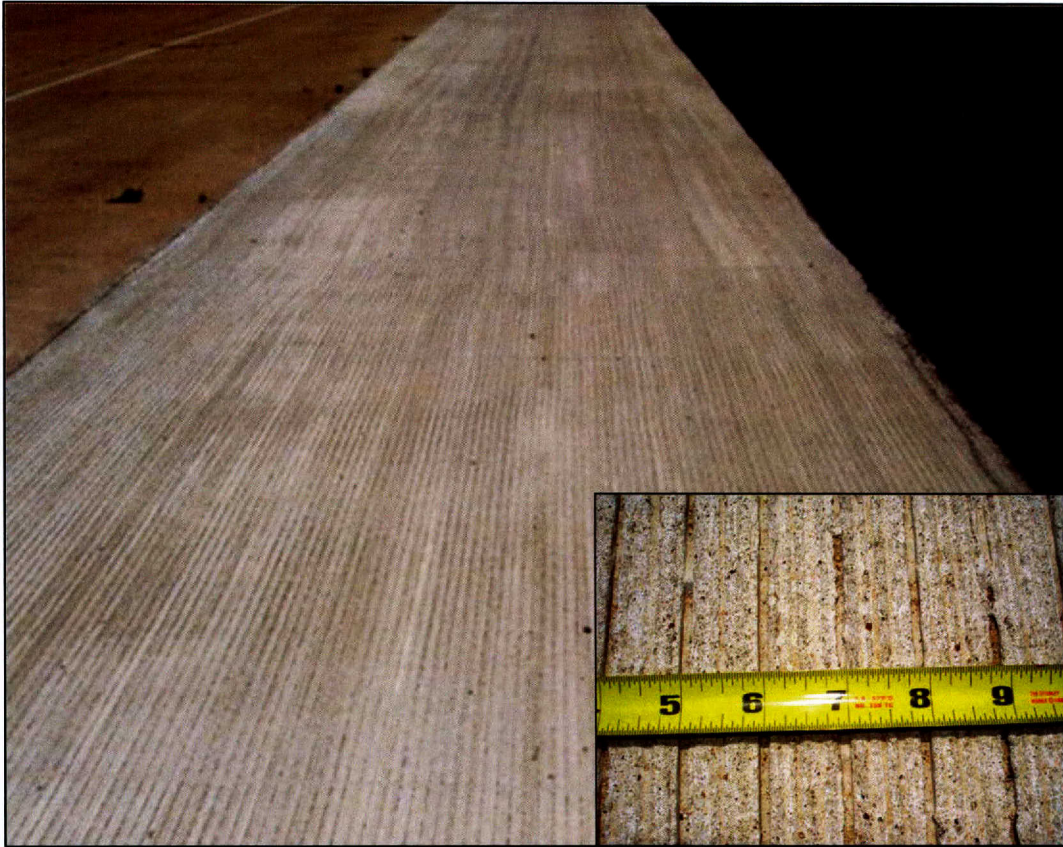
Figure 51. One-inch Longitudinally Tined CRCP Section.
