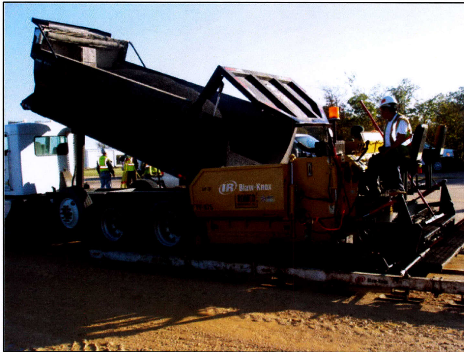
Figure 31. Paving Machine Used to Place Type C Mix.
