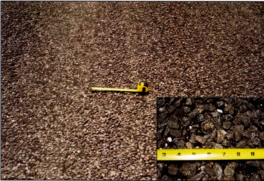
Figure 56. Grade 3 Chip Seal Section.
