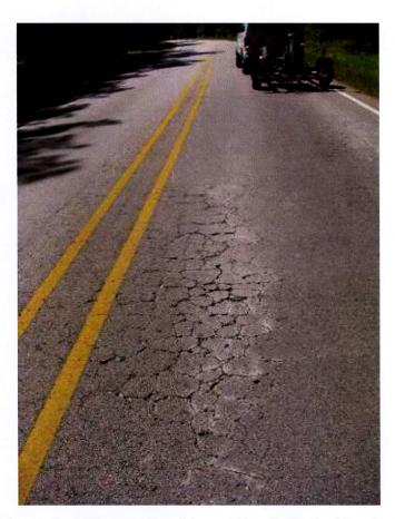
Figure 8. Alligator Cracking at South End of Project.
