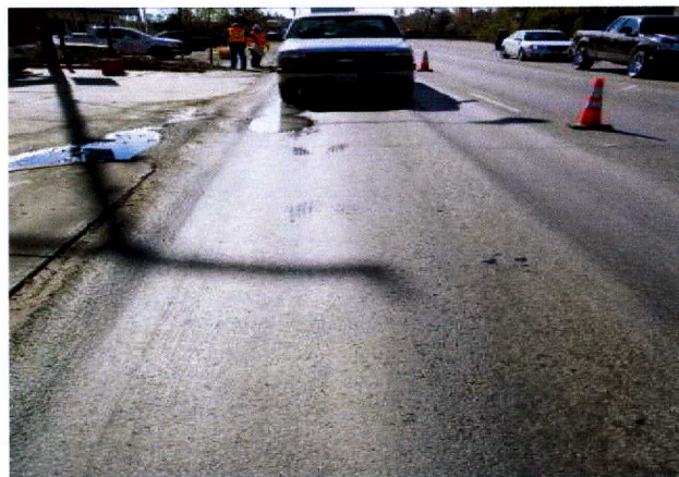
Figure 1-2. Severe Surface Rutting on US 96 in Beaumont District (over 1.5 inches Rut Depth).
